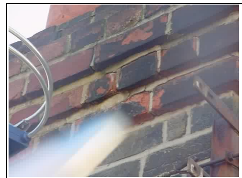
Close up of spalling brickwork
