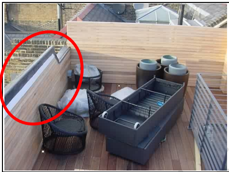
Poor detail, allowing rainwater to drip down the cladding
