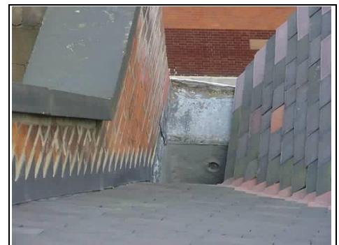
Difficult to access box gutter
