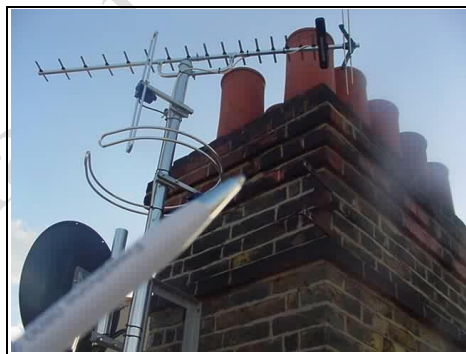
Spalling brickwork
