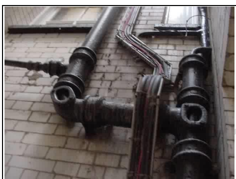
Staining indicates soil and vent pipes are leaking
