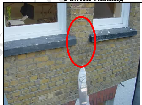
Hairline cracking
