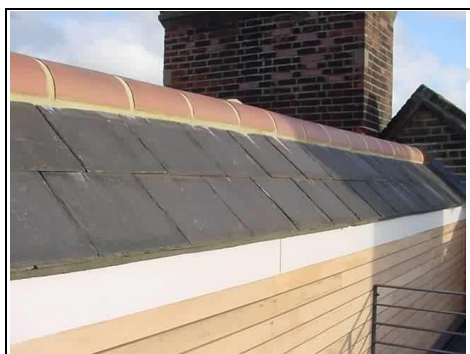
Fascia on terrace has no gutter, without guttering pattern staining will occur
