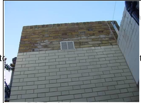
Signs of dampness to central parapet walls
