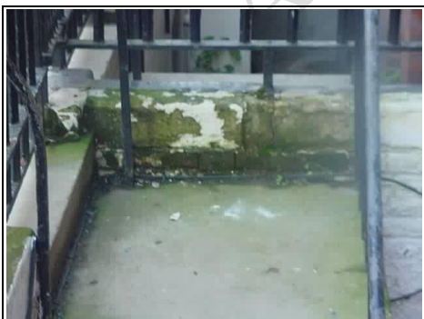
Dampness at top of external area
