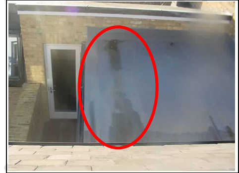
Ponding on single ply roof
