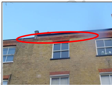
Appears to be deterioration to the red brickwork indicating that the gutter above may be leaking onto it.
