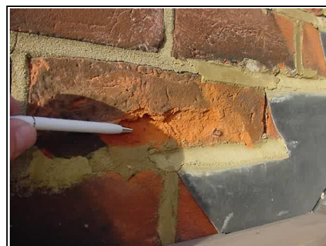
Spalling brickwork
