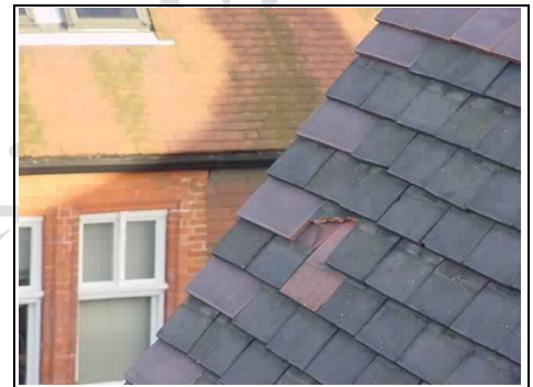
Broken and undulating tiles
