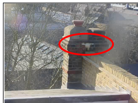
Cement mortar pointing
