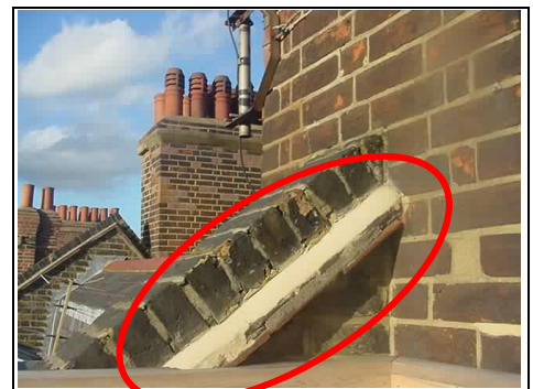
Inappropriate cement repointing
