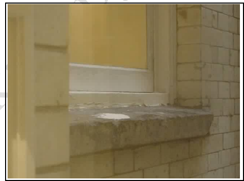
Window facing central void requires painting to window and window sill.
