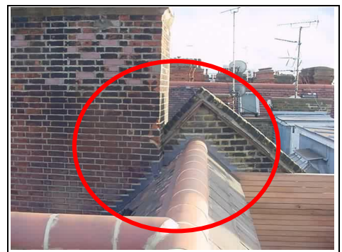
Awkward detail where chimney meets the roof
