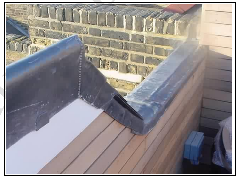
Poor detailing on terrace roof
