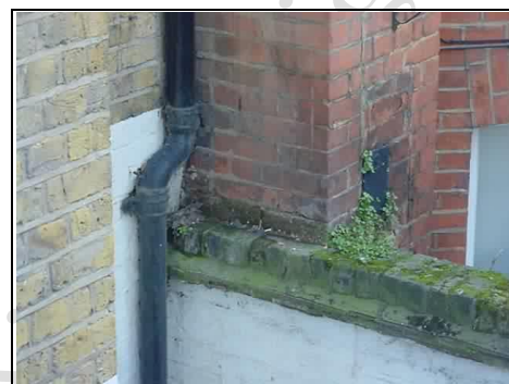
Leaking downpipe
