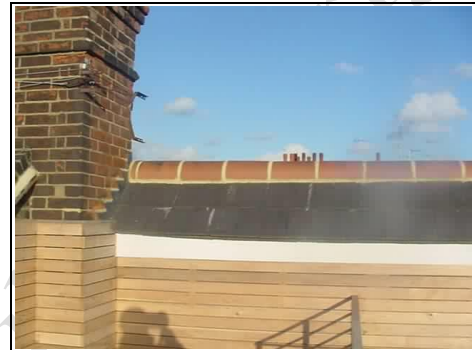
Poor detailing where water will run down the timber and cause pattern staining we believe
