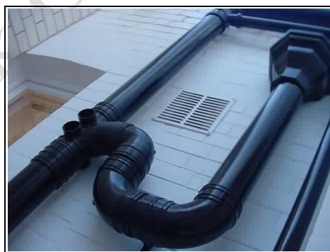
New plastic soil and vents pipes and guttering
