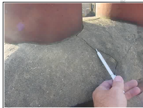
Crack to cement haunching
