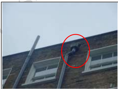
No lead behind hopper head
