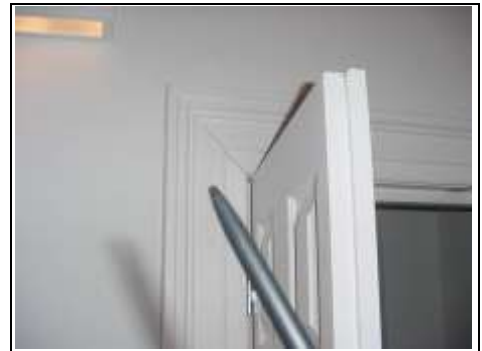
Cracking around entrance door to drawing room, Apartment Four
