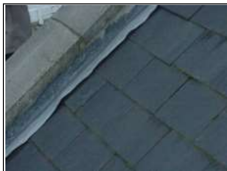
Lead flashing is lifting
