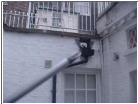
Hopper head left hand side wall of Apartment Two
