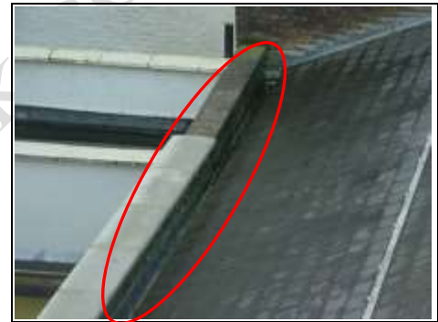
Awkward box gutter that we believe is leaking
