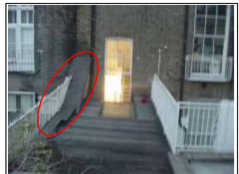
Rear right hand side parapet wall has been completely tarred
