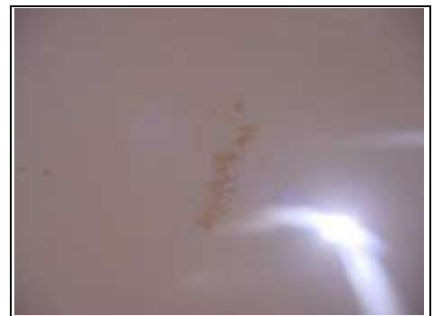
Dampness coming into the ensuite from the kitchen above in Apartment Two
