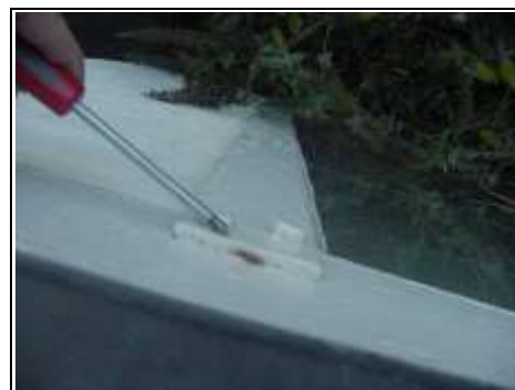
Rusting to metal work on timber windows
