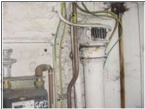
Vent for deep sewerage drainage
