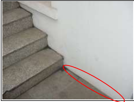
Poor render detail- this is why there is dampness in the property
