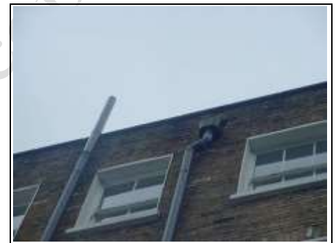
Hopper head taking water off the roof
