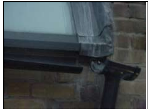
Guttering is broken
