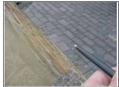
Hairline cracking.
