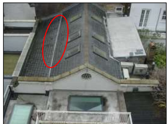
Rear pitched roof Awkward box gutter (red)
