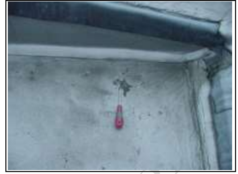
Solar reflective paint is wearing away
