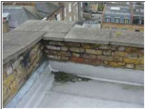
Rear parapet wall with paviour slabs to the top
