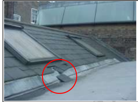
Slates displaced
