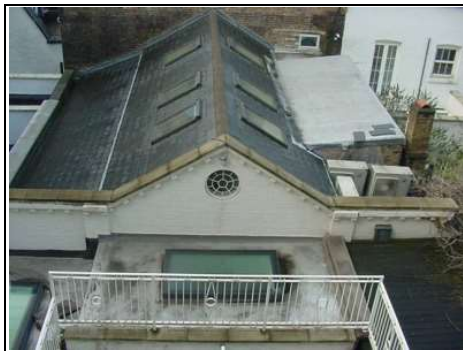
Roof windows to rear pitched roof
