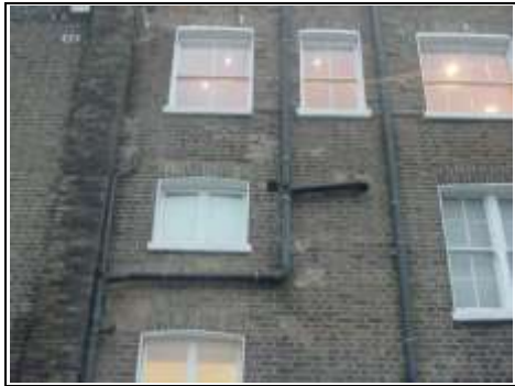
Sash windows to the rear of the property look in reasonable condition
