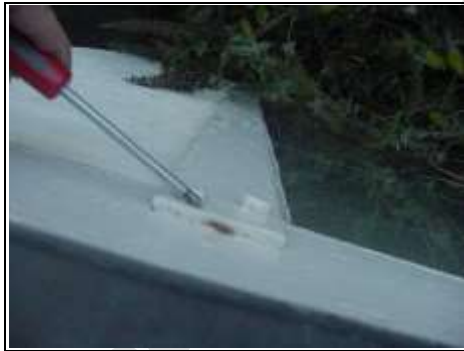
Rusting to the metal work on the timber windows to the right hand side of Apartment Two
