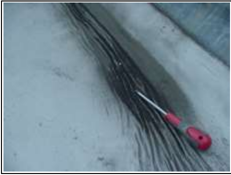
Rucking to the flat roof over Apartment Two
