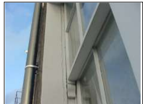
Hairline cracking to render on the reveals of the windows
