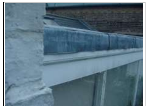
Poor detail requires a gutter, assuming it is not hanging over next doors property
