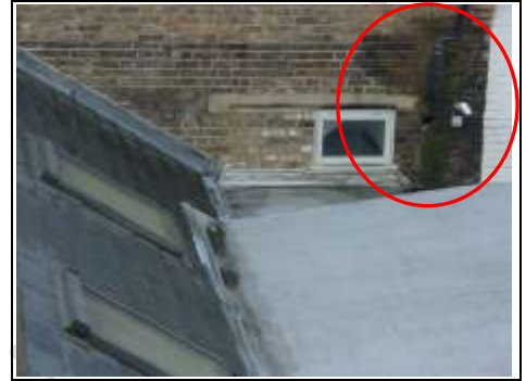
Neighbours gutter leaking onto your wall
