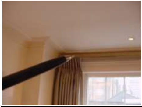
Damp staining at window
