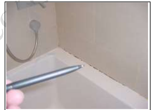
Condensation in bathroom Apartment Three
