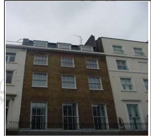
Flemish bond brickwork
