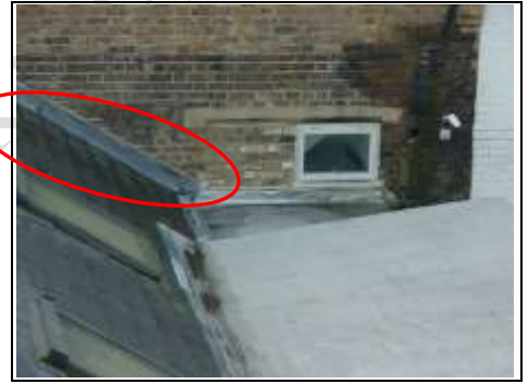
Straight line flashing to right of rear roof instead of the correct stepped flashing.
