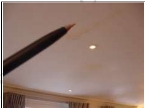
A leak has been painted over in the drawing room in Apartment Five
