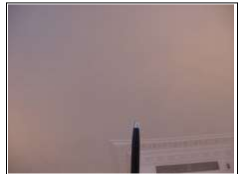
Cracking around the lift area in Apartment Four
