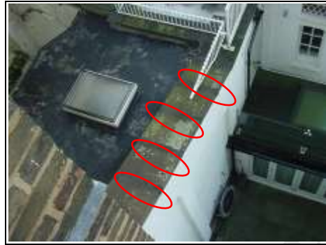
Parapet wall to courtyard has been tarred over the joints
