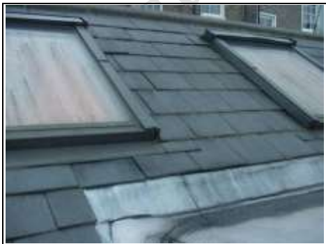
Mould on roof window above Apartment two
