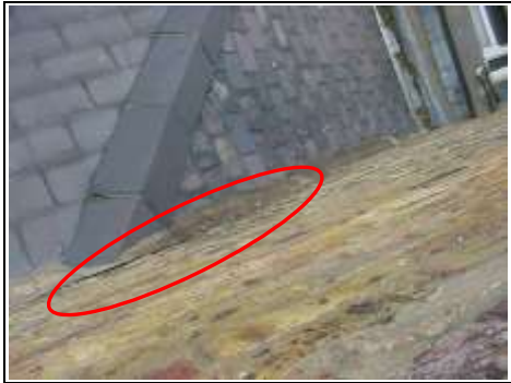
Cracking to concrete fillet
