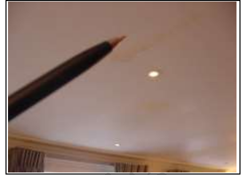
Damp staining relating to the main roof
