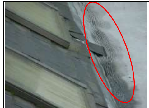
Roof to the right hand side is starting to deteriorate and ruck
