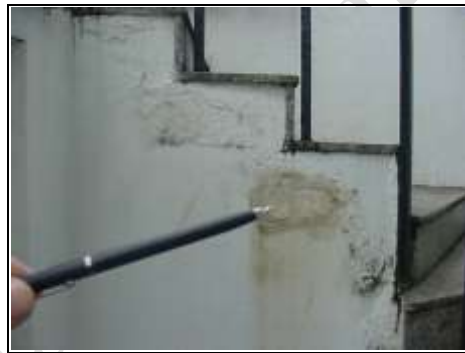
Damp coming from the stairs into the wall. Asphalt tends to be the only way to resolve this
