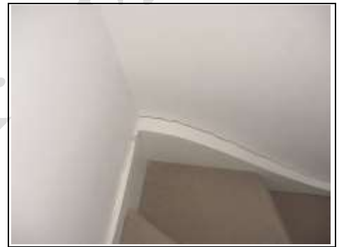
Cracking on stairs in Apartment Two leading down to bedrooms
