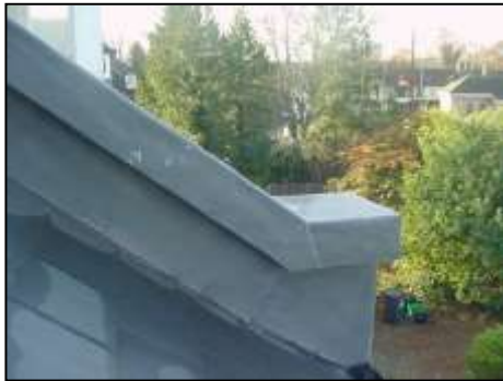
Example of lead capping to a parapet wall on another property.
