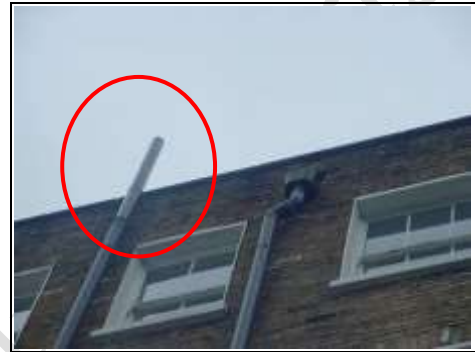
Plastic soil and vent pipe
