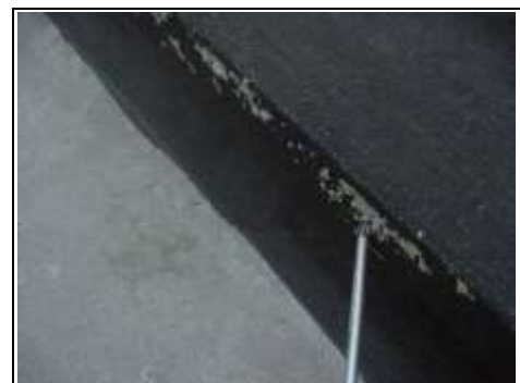
Damage to parapet wall
