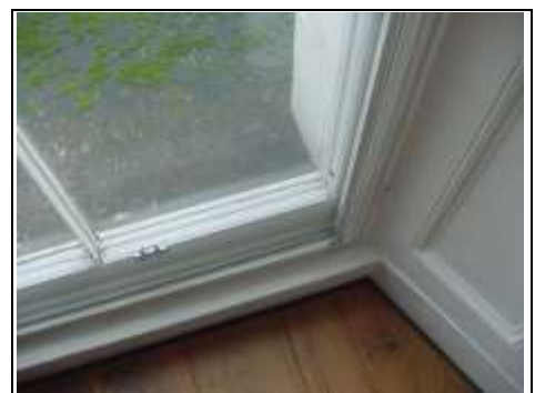
Secondary glazing in Apartment four
