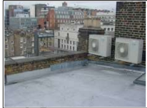
Comfort cooling units on chimney
