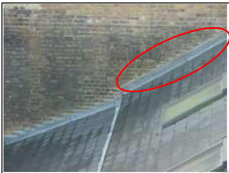
Straight line flashing to left of rear roof instead of the correct stepped flashing.
