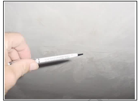
Hairline cracking
