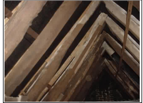
General view of roof
