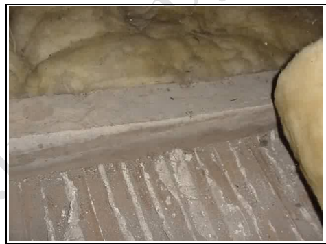
Lath and plaster ceiling
