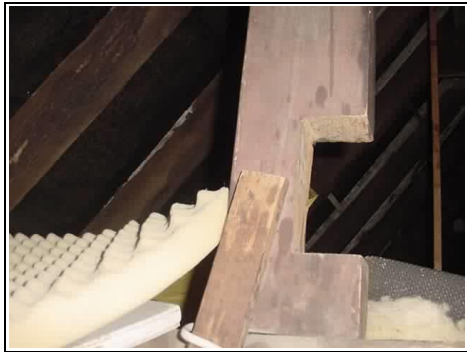
Re-used timber and approximately half of it cut
