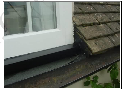
Modern replacement timber window
