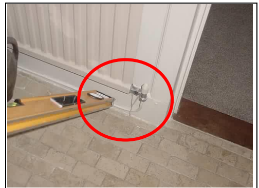
Micro-bore pipes
