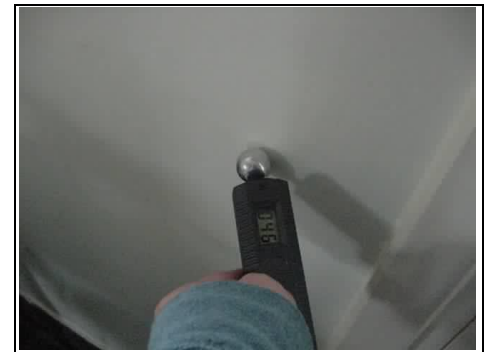
Testing for rising damp
