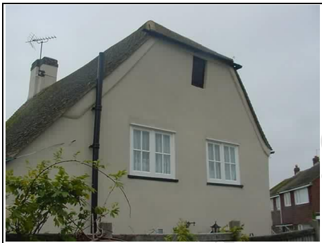
Thickening of the render at high level
