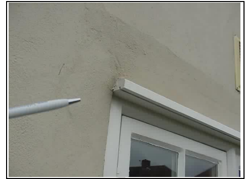
Drip detail to window
