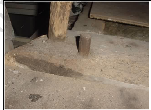
Peg fixing spine beam not tied in
