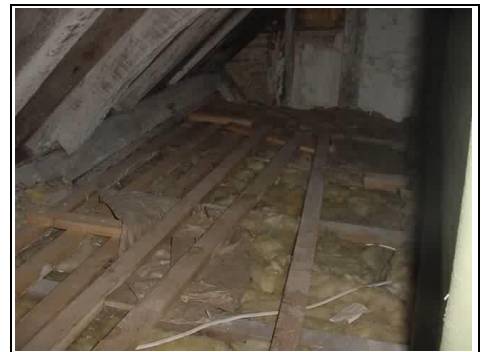
Back to backing of timbers
