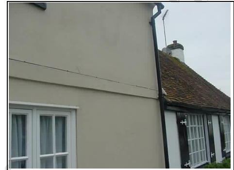
Painted cement rendered walls covering timber frame
