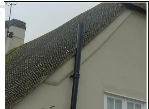
Soil and vent pipe to left of property
