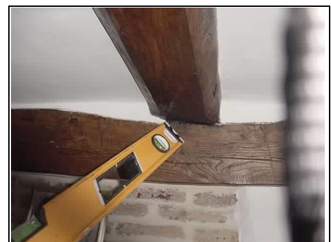
Spine beam that does not tie in
