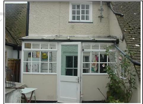
Rear low level roof
