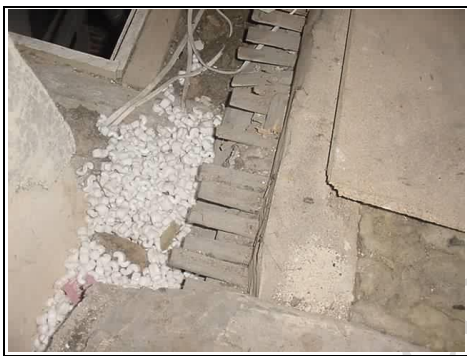
Lath in ceiling overlaid
