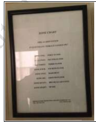
Zoning for fire alarm system which is what we always recommend
