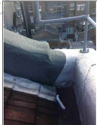
Mineral felt to rear parapet wall
