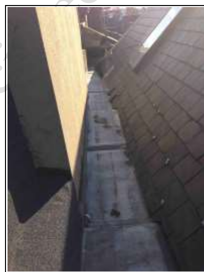
Main roof to left hand side
