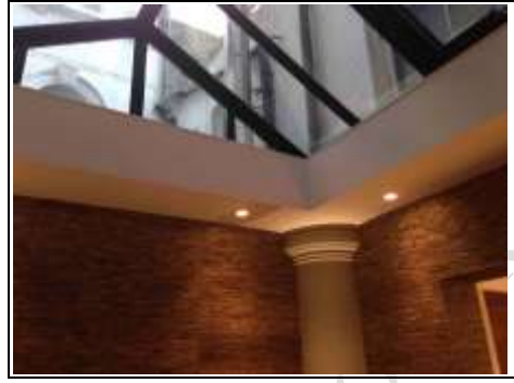
Looking up at glass roof
