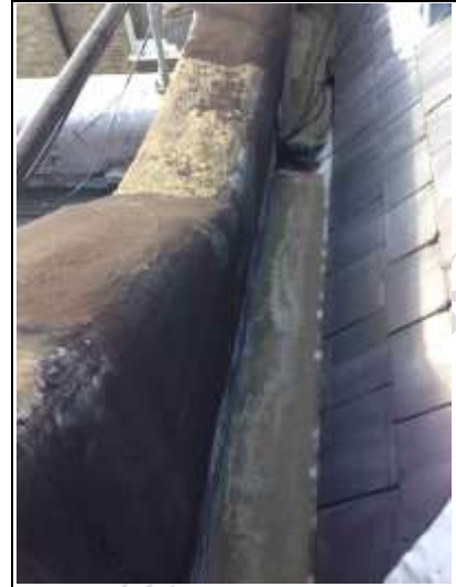
Bitumen covered parapet wall
