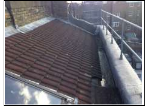
Single pitched concrete tiled roof
