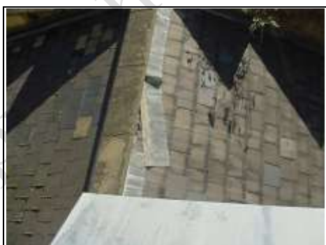
Parapet wall on rear pitched roof
