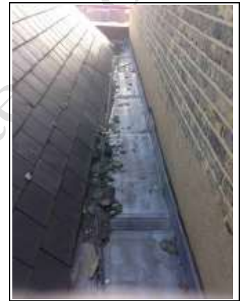
Stepped box gutter to right hand side of main/loft conversion roof
