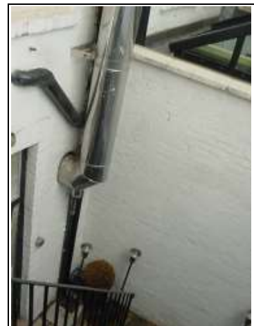
Painted brickwork at low level
