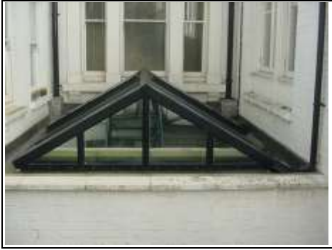
Glass covering of void
