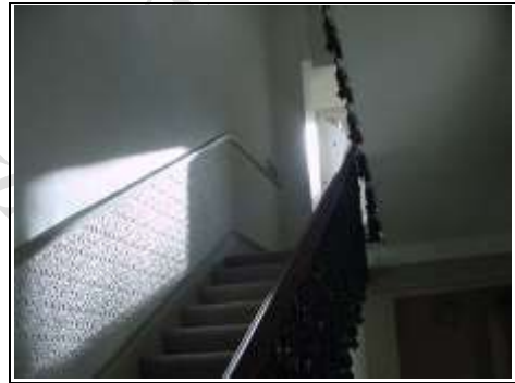
Shared stairway / fire escape
