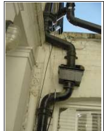
Cast iron hopper head
