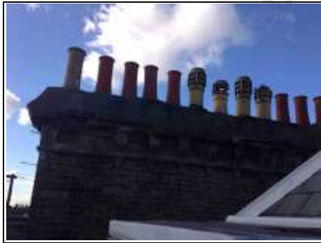
Chimney to front right
