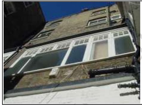
Rear of property from middle void
