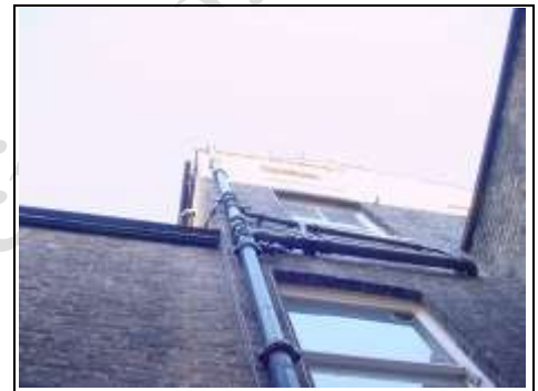
Looking up at the brickwork
