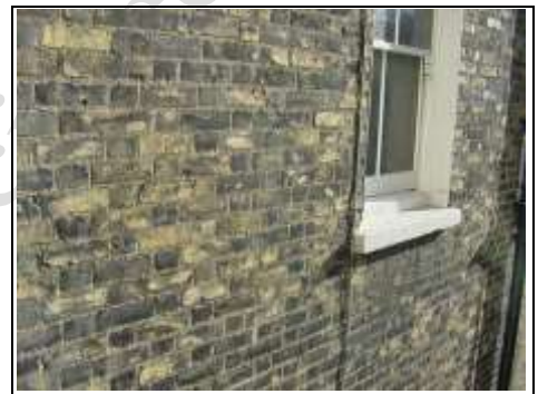
Flemish Bond brickwork at high level
