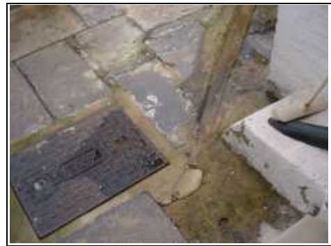
Manhole in middle void
