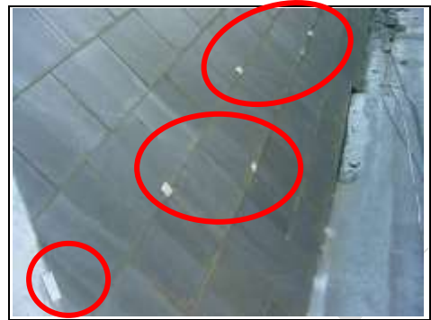
Lead tingles to manmade slate loft conversion roof
