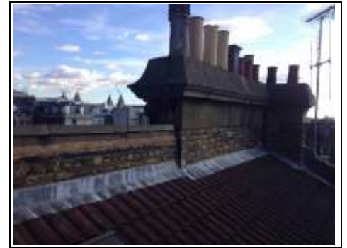
Chimney to rear left side
