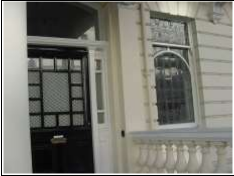
Shared front entrance door
