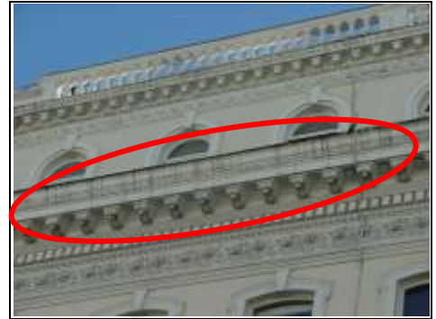
Balustrade and ledges
