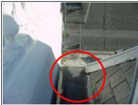
Box gutter to front
