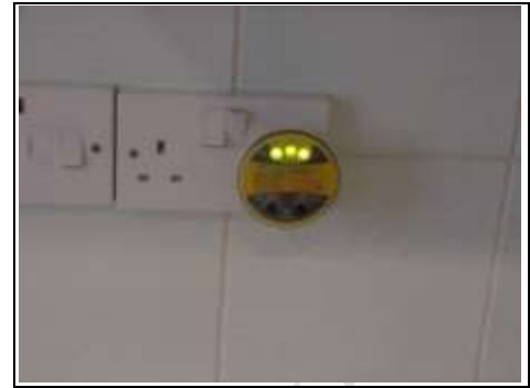
Earth test taken in ground floor kitchen
