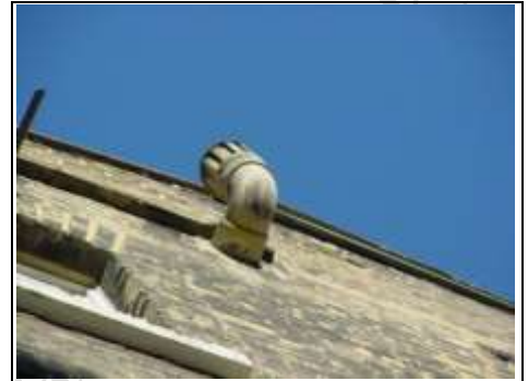
Asbestos flue to rear
