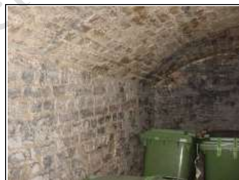
Vault under road
