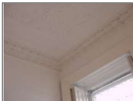
Over painted moulding on ground floor
