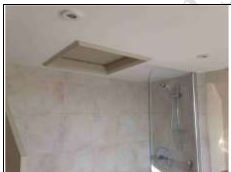
Access hatch in bathroom
