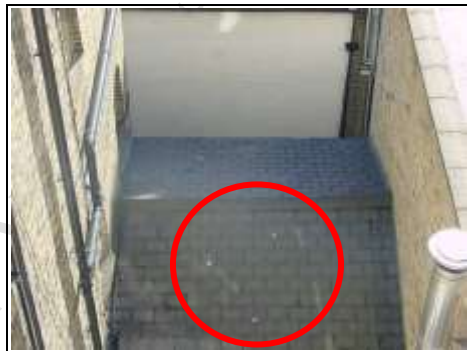
Lead tingles on double pitched lead roof to rear
