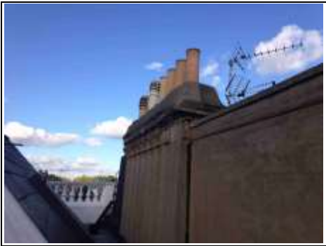
Chimney to front left side
