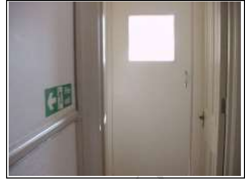
Fire exit to rear of ground floor
