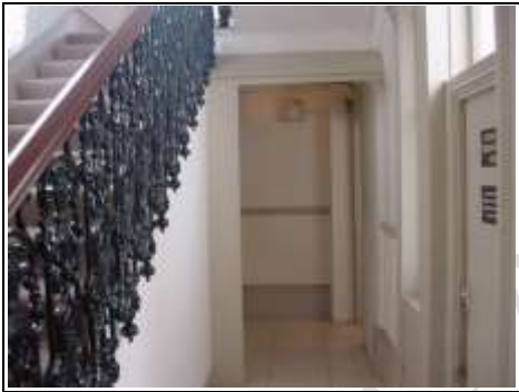
Shared entrance hall and staircase
