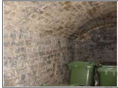
Vault under road currently being used as a bin store
