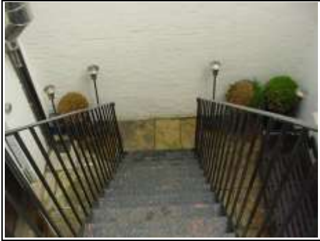
Fire escape stairs
