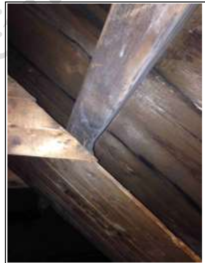
Vertical close boarding, we normally see this horizontally
