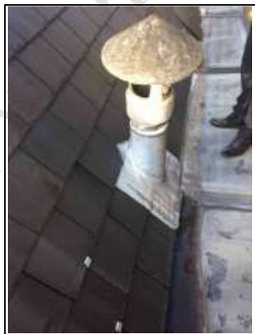
Asbestos flue to main/loft conversion roof on left hand side
