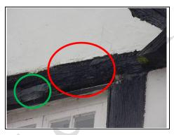
Hole above the window in gable end wall (red) Cement or plastic repair (green)
