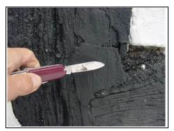
Plastic wood repairs to the timber structure
