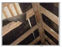
Quartered timber with bark left on in left side roof. Underlayer torn
