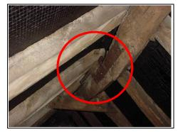
Metal bracket added to broken ridge timber
