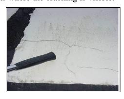
Loose render around the cracking
