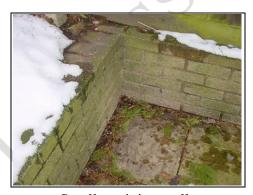
Small retaining walls need weep holes
