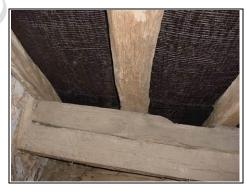
This photo shows the common rafters in the left hand side (the ones that form the pitch of the roof) and the dark area between is the underlayer
