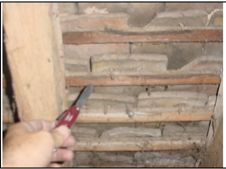
Underside of peg tiles right side roof
