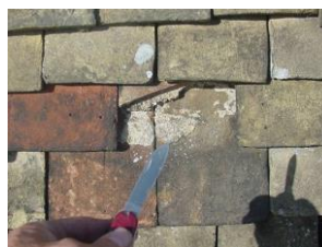
Broken and missing tiles
