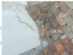
Disintegrating tiles
