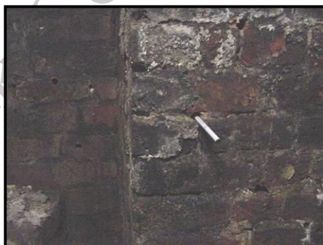
Pen indicates an example of one of many holes drilled in the wall in the basement
