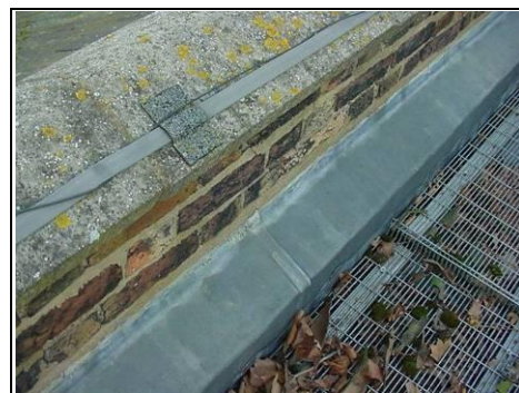
Parapet wall has been wrongly repointed in cement mortar
