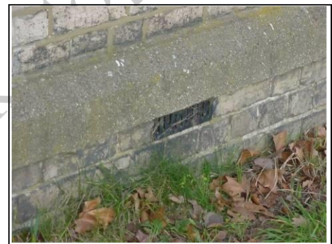
Airbricks that lead into cellar
