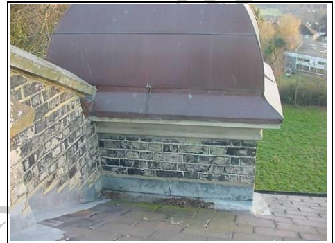
Natural areas due to the way the roof has developed that are awkwardly detailed, such as this one with the rear turret roof being a trap for leaves and water
