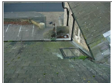
Roof light five – left hand side This is an awkward detail with vegetation growing at the top that needs to be removed as part of your annual maintenance programme
