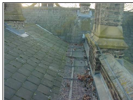
General view of roof showing box gutters
