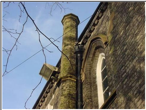
Chimney on right hand gable, overflowing hopper head causing deterioration to brickwork
