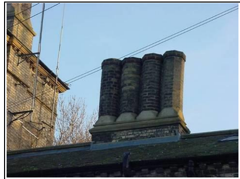
Minor spalling brickwork
