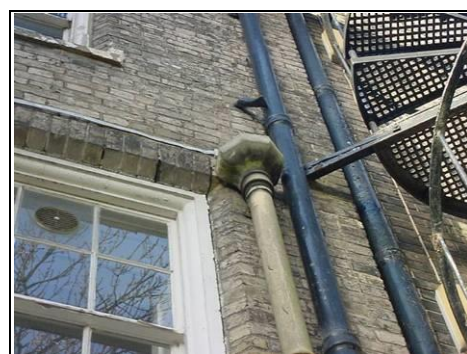
Lead pipework
