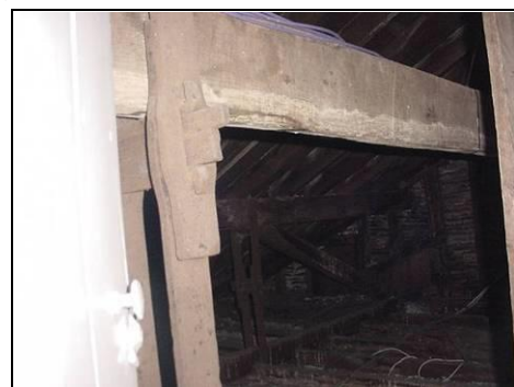
Woodworm to front left hand side roof
