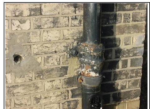
Cast iron downpipe being linked to a plastic downpipe, we assume the original cast iron has rusted away
