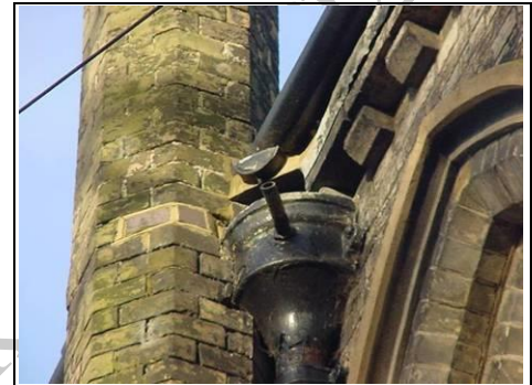
Hopper head overflowing, chimney needs repointing
