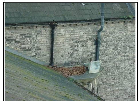
Oriel flat roof right hand side which is leaking
