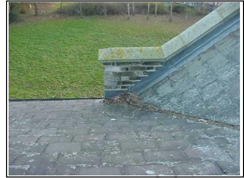
Ongoing maintenance battle against the leaves and branches blocking the gutters up on the roof
