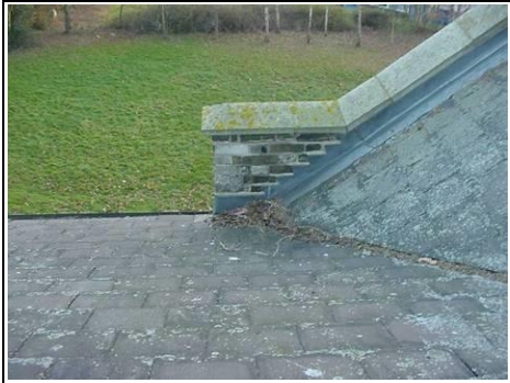
Blocked valley gutter
