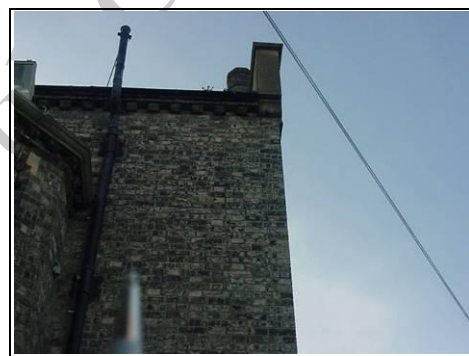
Vertical cracking to right hand wing
