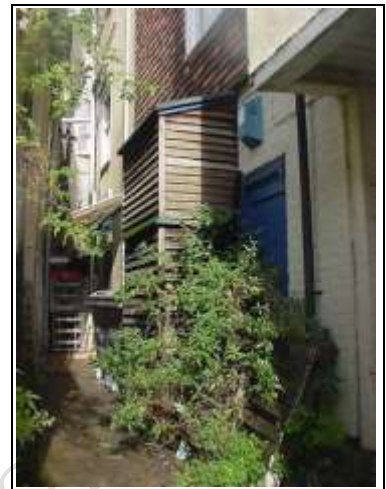
Rear view- shiplap boarding needs re-staining
