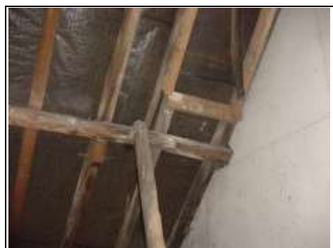
Pole timbers and some wooden pegs
