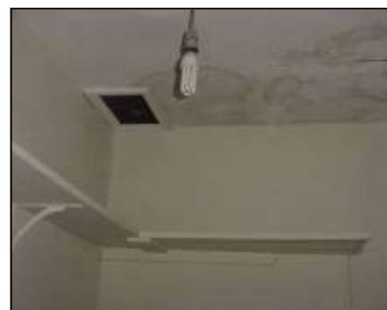
Dampness above staircase area
