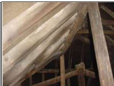
Cut timber roof
