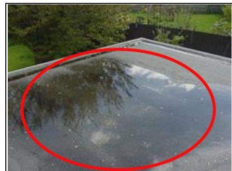
Example of ponding on a flat roof
