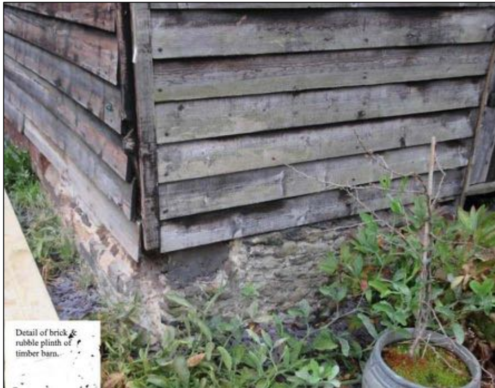
Detail of brick rubble plinth of Timber Barn
