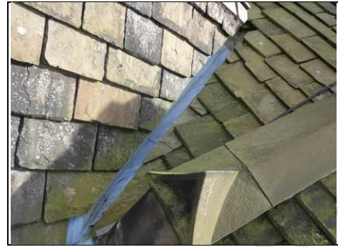
Repairs to valley gutters Aerial view – 360 photo
