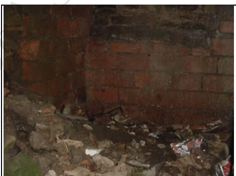
Close up of brickwork at end
