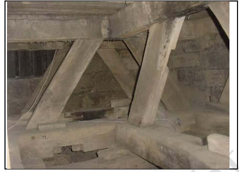
Timberwork in the old Bell Tower
