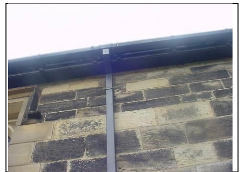
Gutters and downpipes
