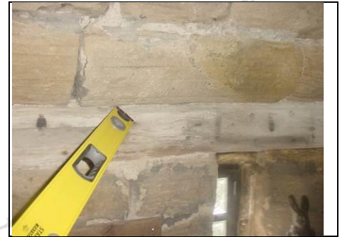
Timber Wooden lintel
