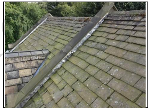
Flashband repairs on parapet
