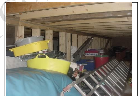
Underneath lounge floor
