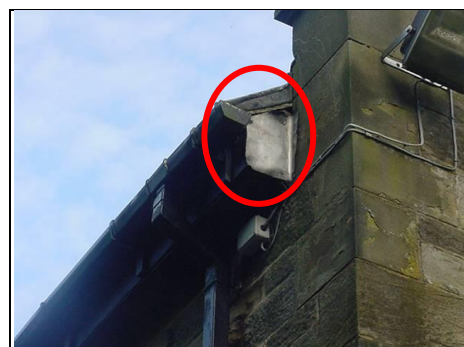
Flashband repair front right side
