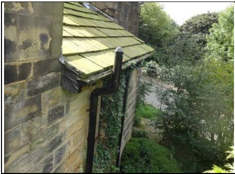
Soil and vent pipe to rear left
