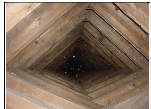
Looking down scissor roof over Nave
