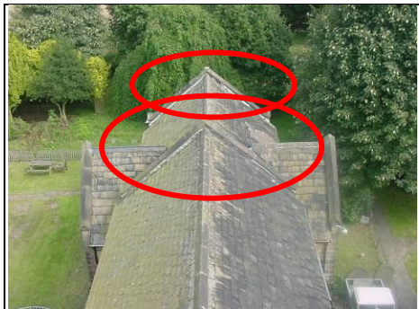
Parapets to nave and chancel
