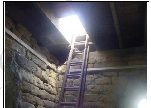
Access to tower roof from Belfry
