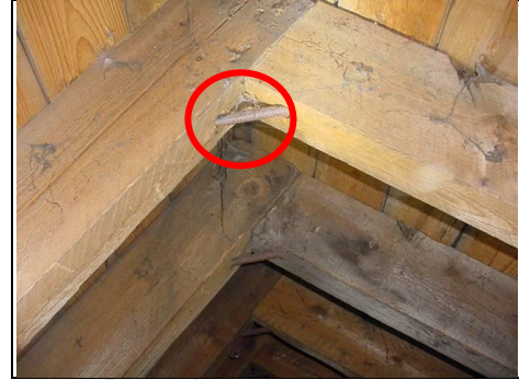
Close up of metal tie bars
