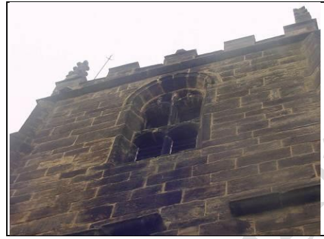
High level windows to Tower
