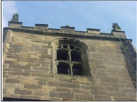
High level windows in tower
