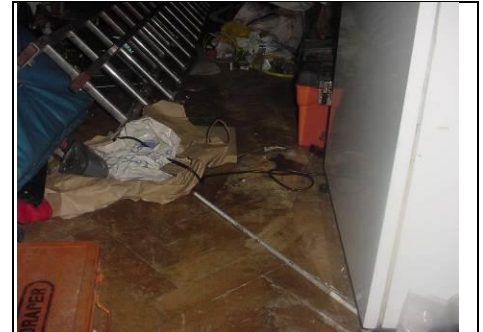
Old parquet flooring
