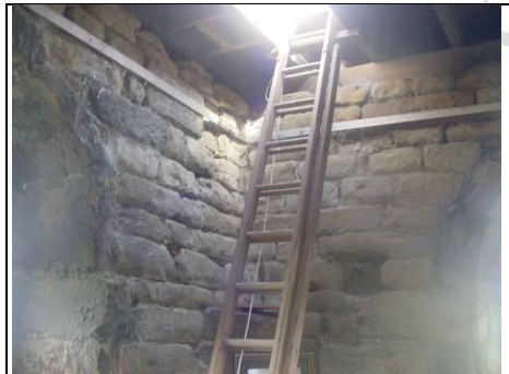
Bracing running around the top of the Tower
