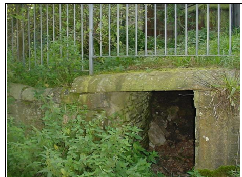
Close up – sealed by brickwork
