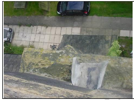
Rainwater discharging from tower flat roof via lead gully
