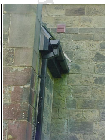
Flashband repair to fascia on north side
