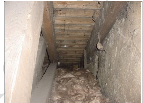
Close boarding and insulation
