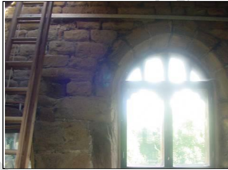
Window and ladder to roof
