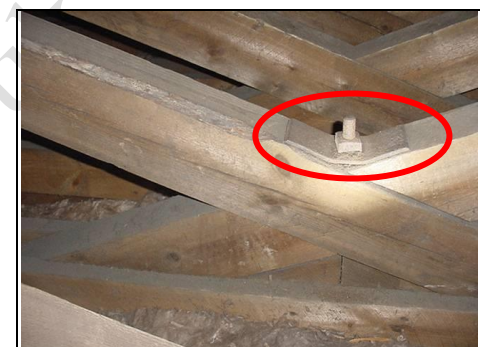
Bolt at top of horizontal tie bar
