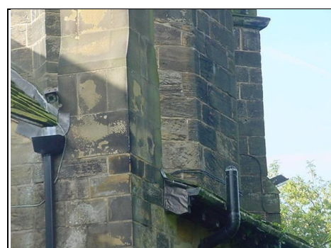
More Flashband repairs
