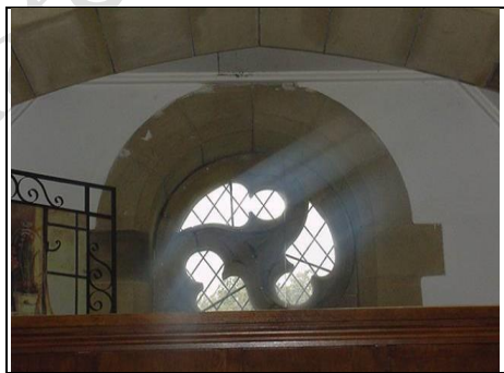
Curvilinear window internally
