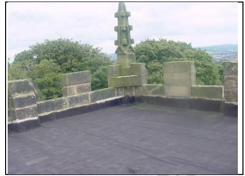
Repairs have taken place to the Tower parapets
