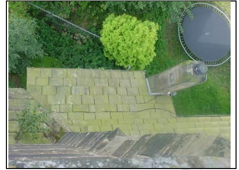
Rear middle roof
