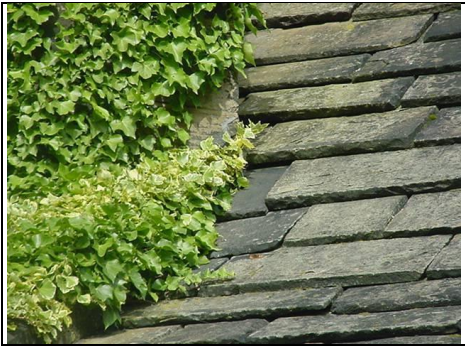
Damaged slabs have been replaced over entrance porch with a thinner slab
