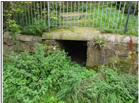
Opening on the roadside
