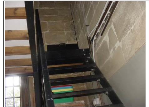
Metal stairs to first floor
