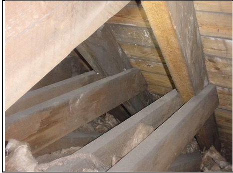
Substantial timber trusses, spaced approx. 350mm apart (not measured)
