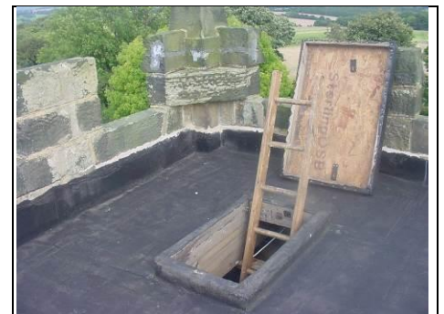
The black felt roof with wooden ladder access
