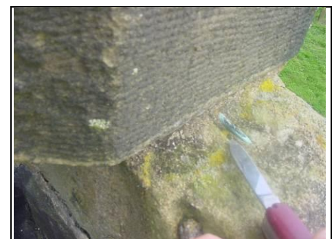
Metal bars tying stonework of battlements/castellations
