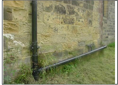
Rear right soil and vent pipe
