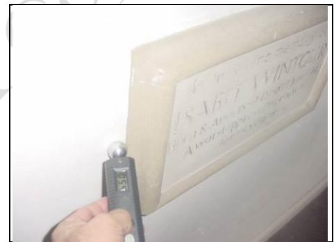
Testing for lateral dampness
