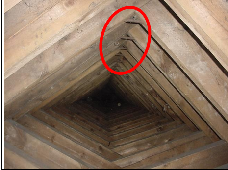
Metal tie bars to ridge
