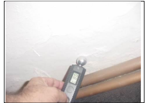
Testing for rising damp
