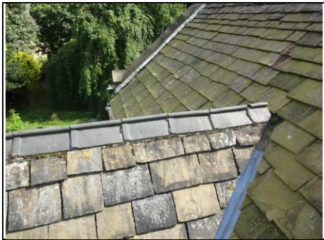
Repairs to valley gutters Aerial view – 360 photo
