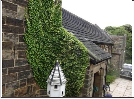
Ivy growing on walls Aerial view – 360 photo
