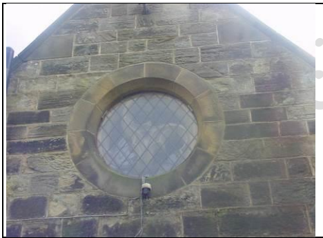
Curvilinear window. We were unable to view this very well due to having a plastic protection on it
