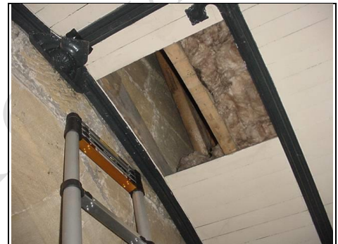
Small access into roof space
