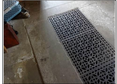
Grill in floor in reception area adjacent to kitchen
