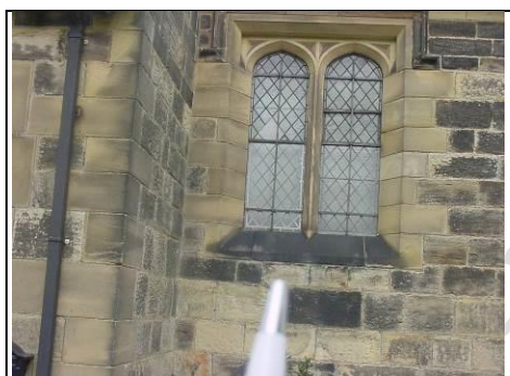
Perpendicular windows to front/south side have been repaired
