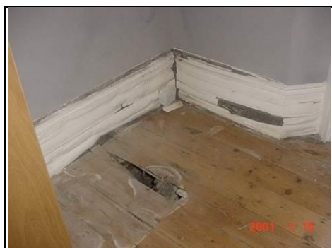
Dry rot example (not this property)
