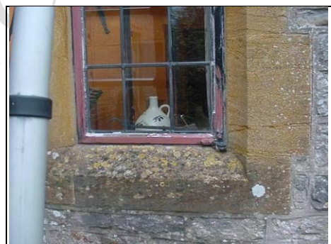
Mullion window with metal casement frame
