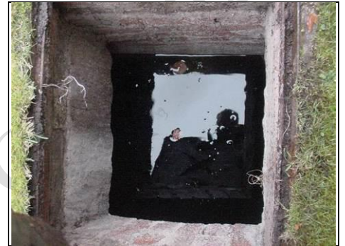
Looking down the well
