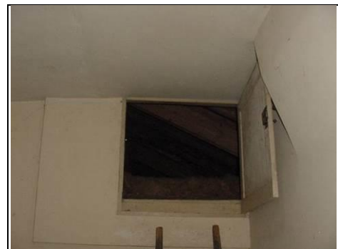
Loft access via half landing
