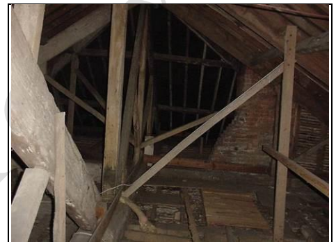
New timbers added
