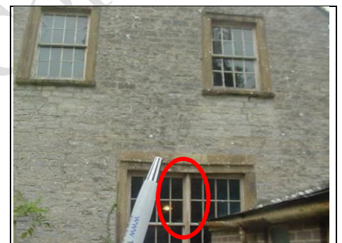
Prop on timber sliding sash windows, set in stone mullions
