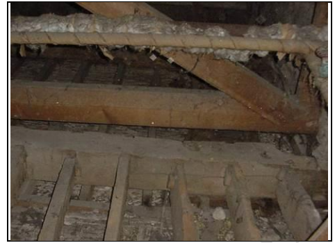
Older timbers to the front of the right side
