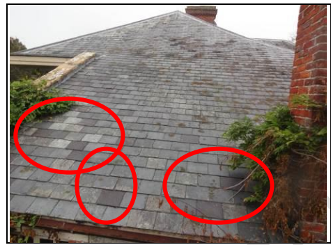
Right side roof Aerial view – 360 photo
