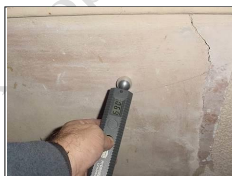
Testing for lateral dampness
