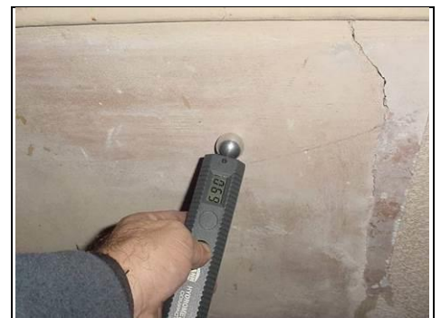
Checking for lateral dampness
