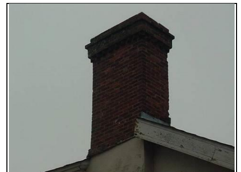
Close up chimney two
