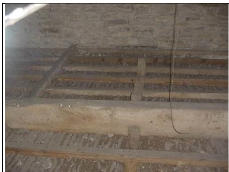
Lath and plaster ceilings viewed from within the roof space
