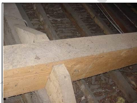
Close up of new timbers
