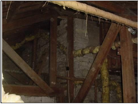
Newer machine cut roof
