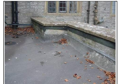
Close up of flat roof and stone parapets
