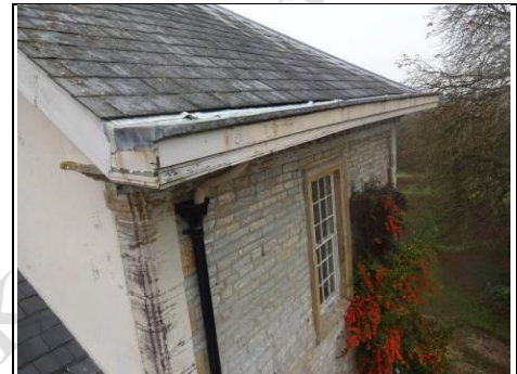
Wide fascias and soffits Aerial view – 360 photo
