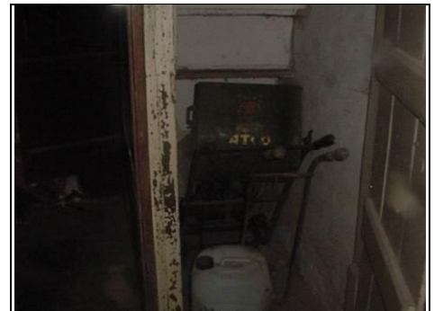
Back of stairs
