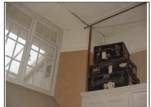
Roof window seen internally within Linen Room
