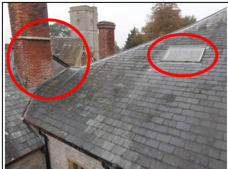
Roof window Aerial view – 360 photo
