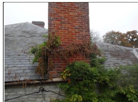
Base of chimney three covered with plants Aerial view – 360 photo
