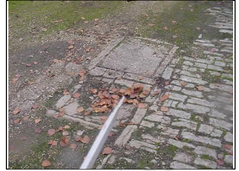
Manhole to right side, we were unable to lift the cover
