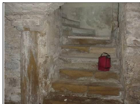
Stone stairs in cellar
