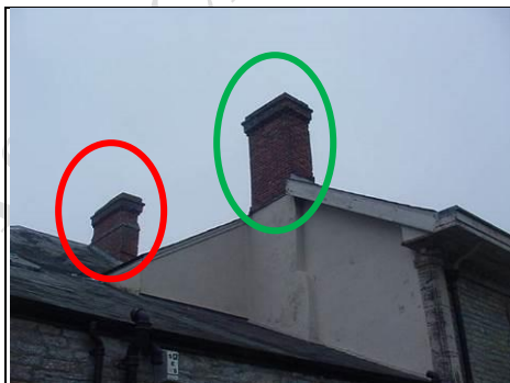
Chimneys one (red oval) and two (green oval)
