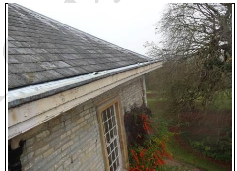
Fascias and soffits and lead detail
