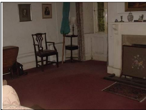
The School Room to the front right is where we believe dry rot is most likely to be
