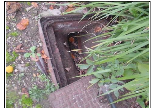
Manhole to front of property
