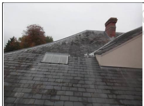
Roof window close to Linen Room Aerial view – 360 photo
