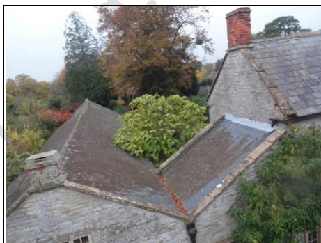
Butterfly roof Aerial view – 360 photo
