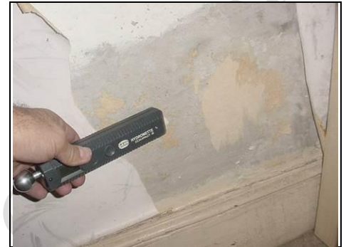
Lath and plaster dry lining / false walling within rear bedroom
