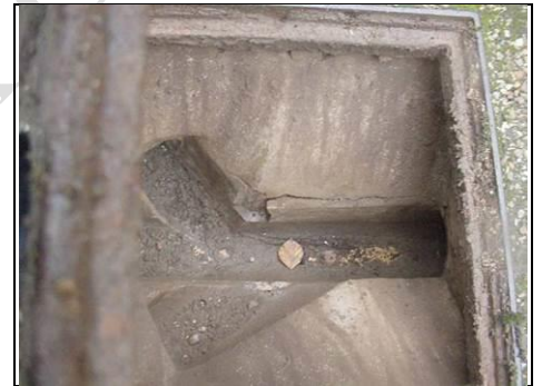
Dry manhole located to the rear near to the kitchen
