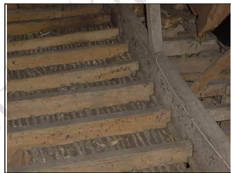
Lath and plaster ceilings, along with ceiling rafters
