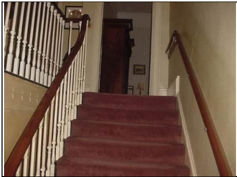
Main house stairs to first floor to right side
