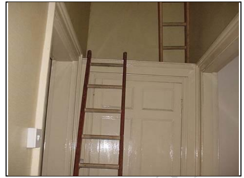
Ladder to roof space on left
