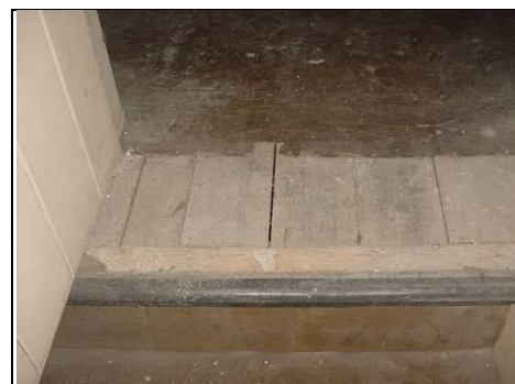
Half landing embedded timbers
