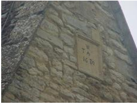
Colleyweston Stone constructed Listed Building
