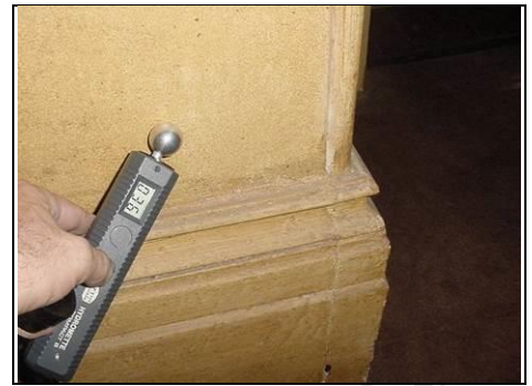
Detailing skirting on to a lath and plaster / false wall
