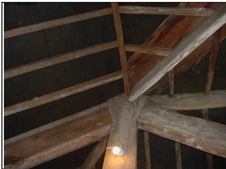
Top of Kingpost roof
