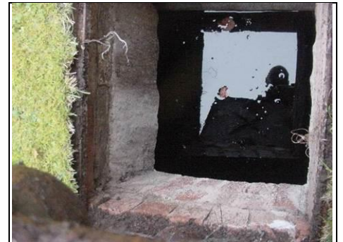
Looking into the well to the rear of the property near the kitchen
