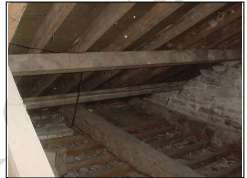
Older ceiling timbers with newer purlin and common timbers
