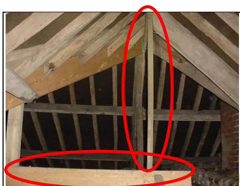
New timbers added to the rear right roof
