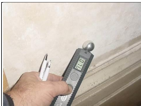
Checking for rising damp
