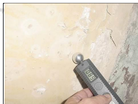
Testing for rising damp
