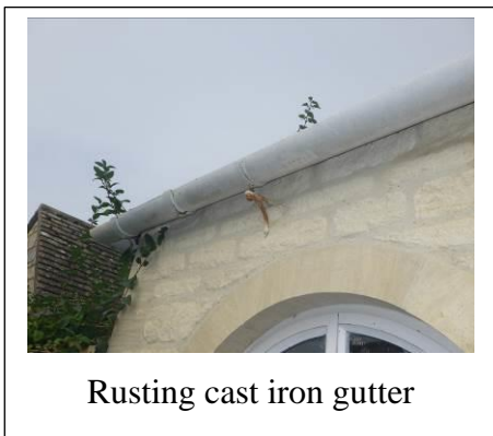
Close up of rusting gutter and fixings
