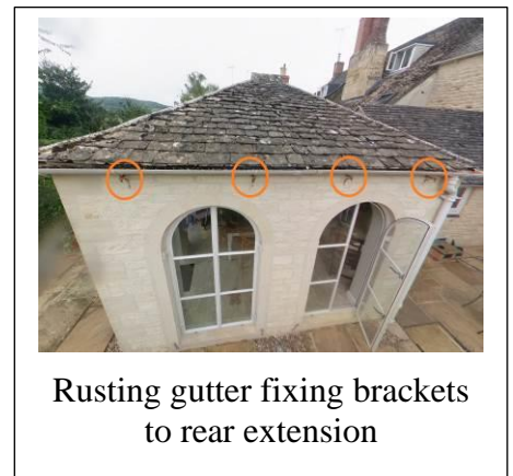
Close up of rusting gutter and fixings
