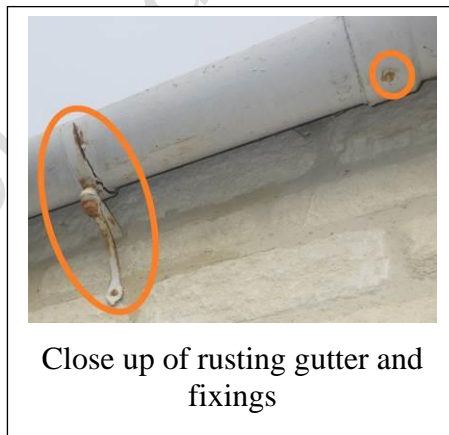
Rusting gutter fixing brackets to rear extension
