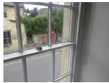
Single glazed timber sliding sash window
