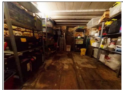
Cellar under kitchen floor
