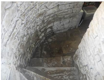
Spiral stairs to cellar
