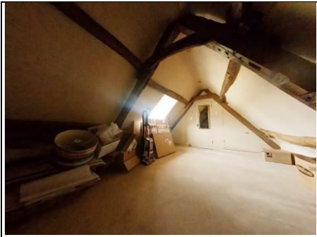
Room in roof from top of stairs
