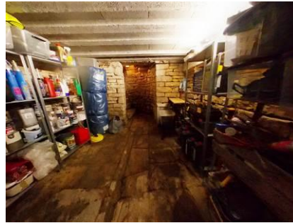
Cellar, no sump pump noted
