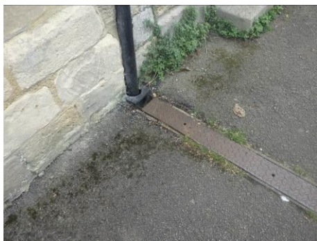
Downpipe going into drain to front
