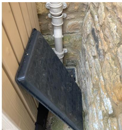
Downpipe to back
