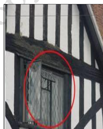
Old style diamond panel lead light in cast iron window opened to air room
