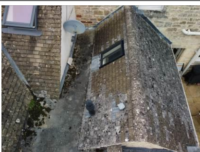
Rear pitched roof, giving extra head height in kitchen
