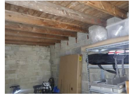
Stonework and timber roof
