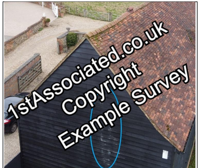
Overflow has overflowed from tank and discharged down building ~ Aerial View - 360 Photo ~
