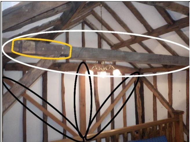
New pegs (yellow) Re-used timber (white) New structural timbers (black)
