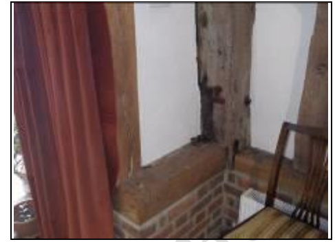
Replacement sole plate or sill boards
