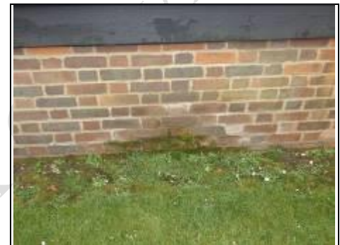
Leaking gutter
