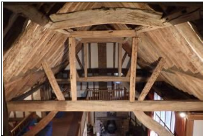
Queen post roof structure ~ Aerial View - 360 Photo ~
