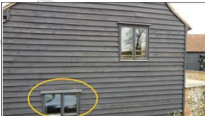
Plastic window to gable end ~ Aerial View - 360 Photo ~
