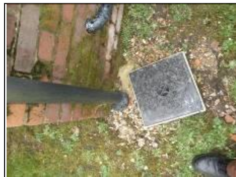
Downpipe and rodding eye to cat slide roof right side
