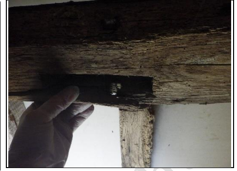
Checking for dampness
