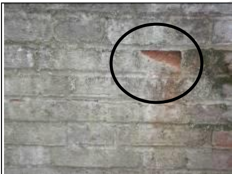
Spalling brickwork
