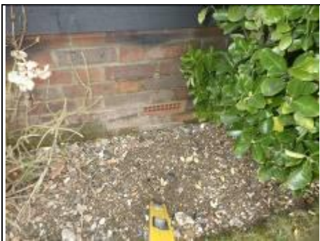
Soft red bricks repointed with a cement mortar
