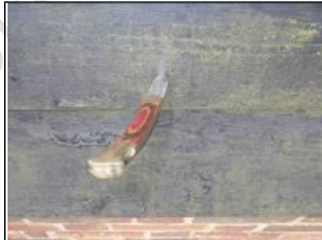
Knife test to weatherboarding
