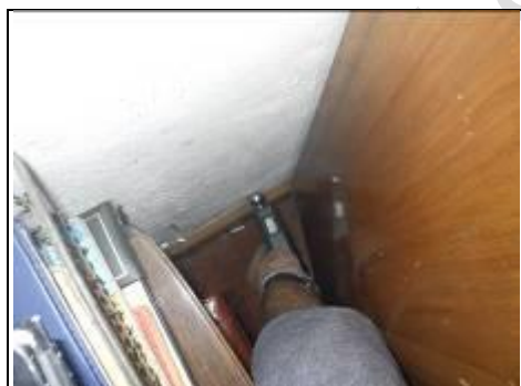
Dry lining in left hand ground floor bedroom
