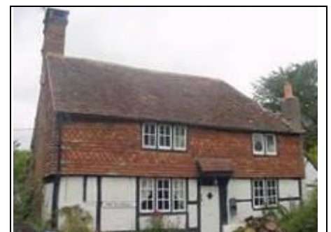
Tudor timber frame property
