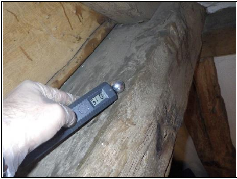
Checking timber for dampness
