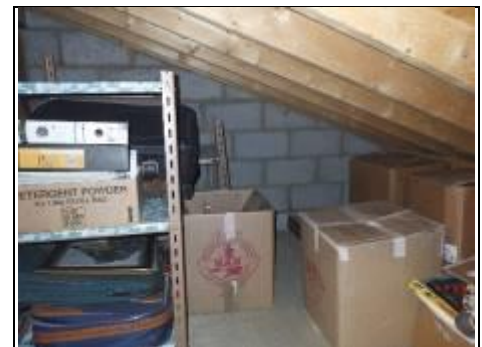
Block work to left hand gable under the cat slide roof
