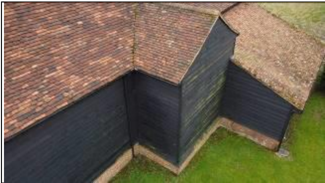
Catslide roof to rear left ~ Aerial View - 360 Photo ~
