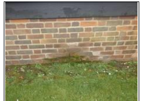
Leaking gutter
