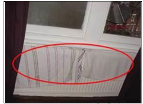
Drying washing on radiators can cause condensation
