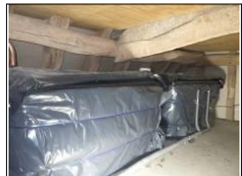
Roof space right hand side
