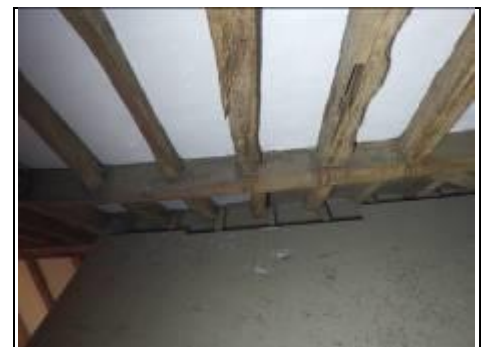
Common rafters into purlin out of true/ movement occurring
