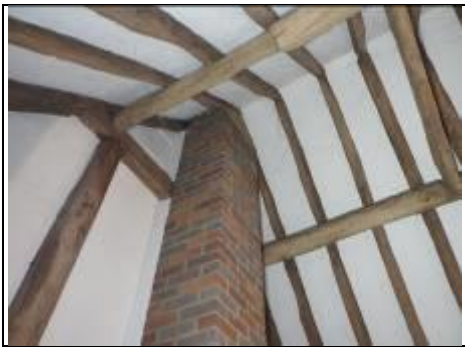
Exposed timber beams at high level and chimney
