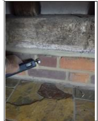
Checking for dampness beneath timber sole plate sill board
