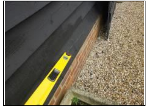
Angle timber over brickwork would this be better in lead this would need conservation officer's approval
