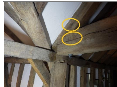
Carpenter's marks visible on timber
