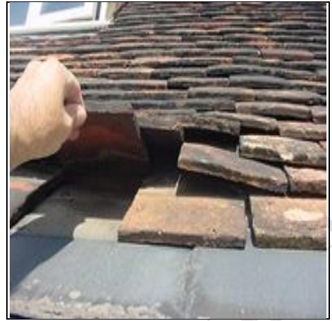
Old peg tiles to Grade II Listed Georgian property roof
