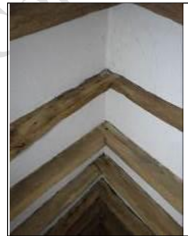
Common rafters coupled at Ridge
