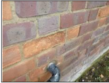
Spalling/deteriorating brickwork
