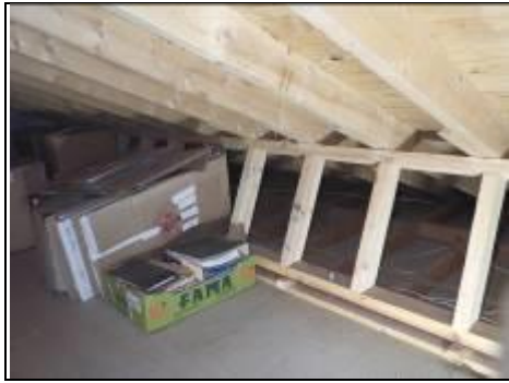
Store under catslide roof
