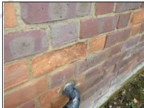
Spalling/deteriorating brickwork
