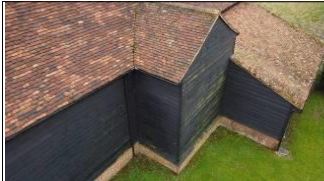
Rear gable end where repairs taken place ~ Aerial View - 360 Photo ~
