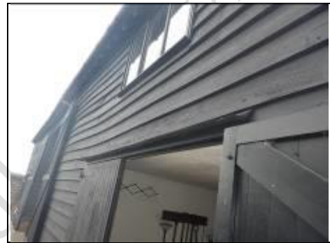
Drip detail to garage door far right
