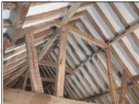
Queen post truss structure with common rafters
