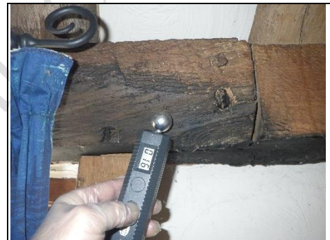
Testing timber for lateral dampness
