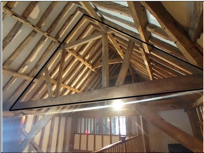
Queen post truss structure ~ Aerial View - 360 Photo ~
