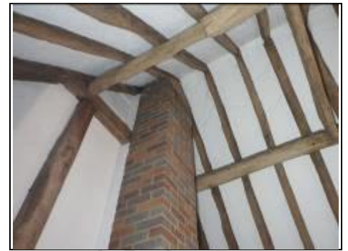
Chimney to right we assume this goes in to the ridge vent
