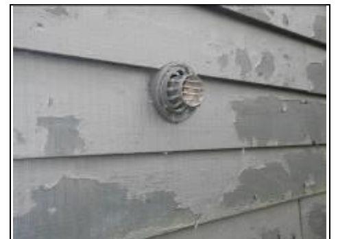
Vent to the rear of the property – why?
