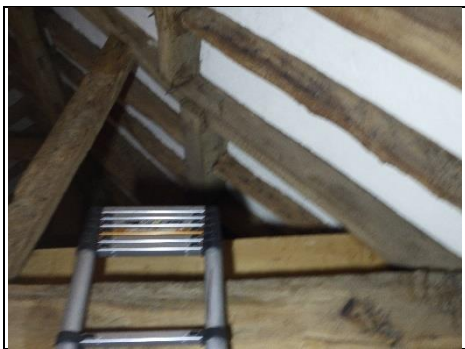
Access to left side
