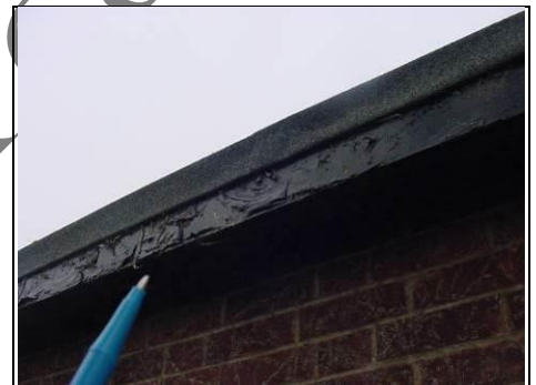
Paintwork blistering to fascias and soffits
