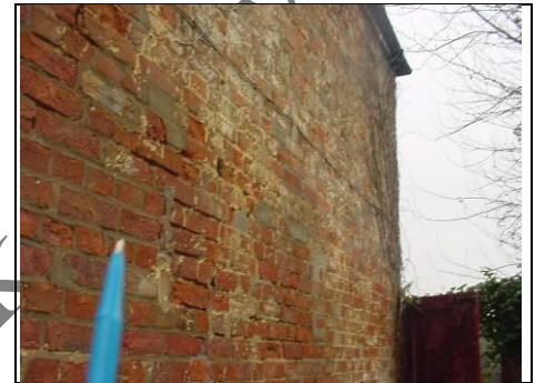
Whole bricks replaced with cement mortar
