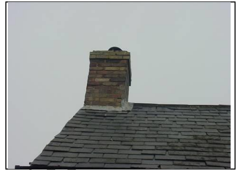
Rear left chimney
