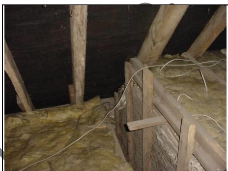
1960's Hessian base underlayer to left side of roof
