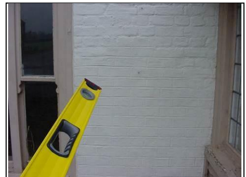
Cement mortar to look like bricks
