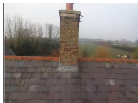
Front right chimney
