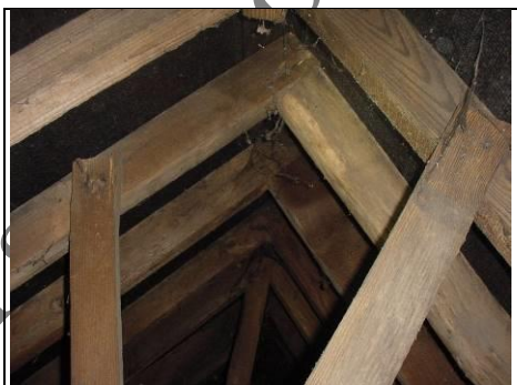
Pegged roof structure in the older original roof
