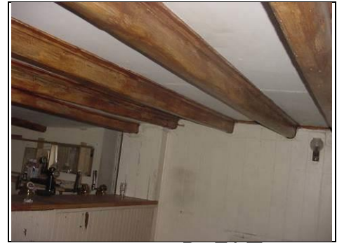
Timber beams to the right side of the main bar
