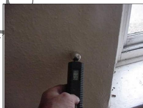
Testing for lateral dampness
