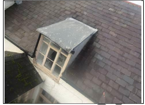
Dormer window Aerial view – 360 photo
