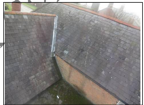
Around 50 lead tingles on main roof
