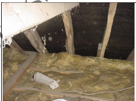
Insulation in the older roof
