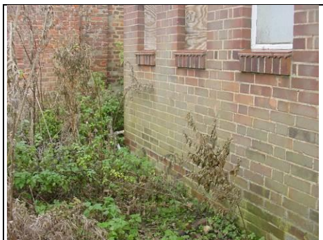
Flemish bond brickwork to rear left
