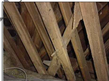
Peg fixings in the roof
