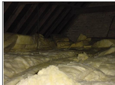
Mass of insulation in the modern roof over the function room
