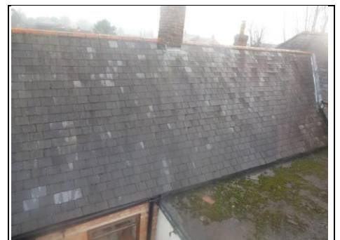
Main roof rear right Aerial view – 360 photo
