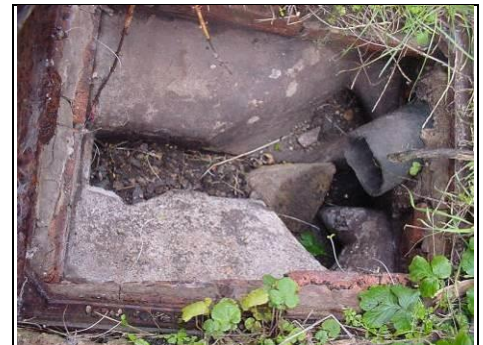
Manhole to the rear
