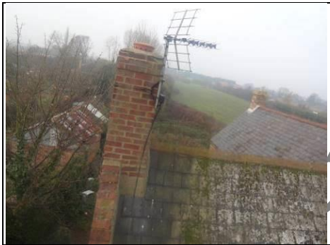
Front left chimney Aerial view – 360 photo
