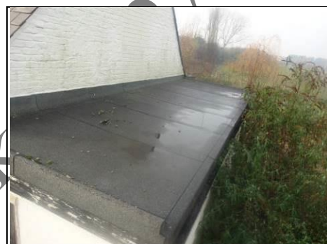
Right flat roof Aerial view- 360 photo
