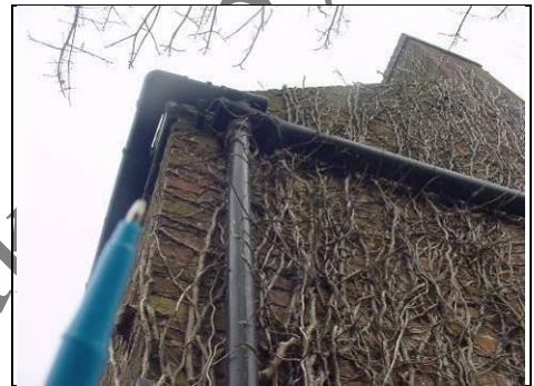
Gutter and downpipe
