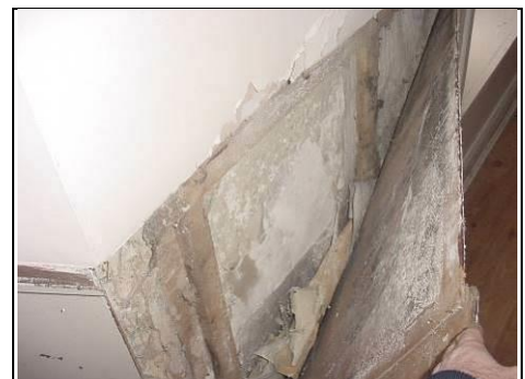
Dry lining internal walls
