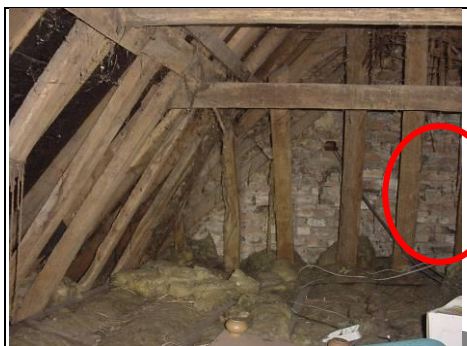
Old roof structure to the left of the property
