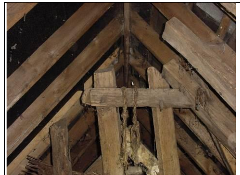
Ridge board in the newer roof
