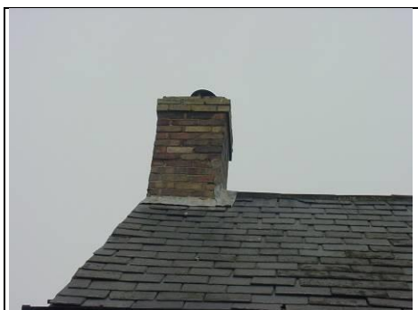
Rear left chimney
