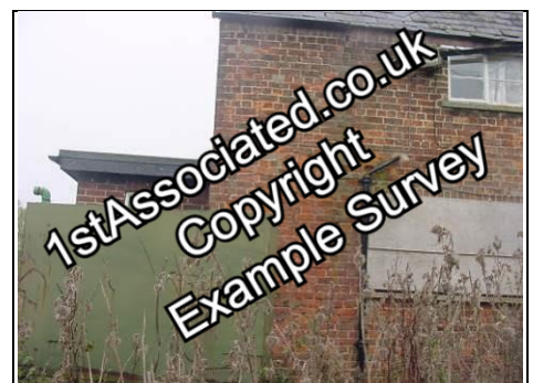
English bond brickwork to the rear
