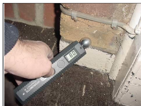
Testing for rising damp
