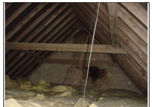
Crack on the front right, hidden within the function room roof
