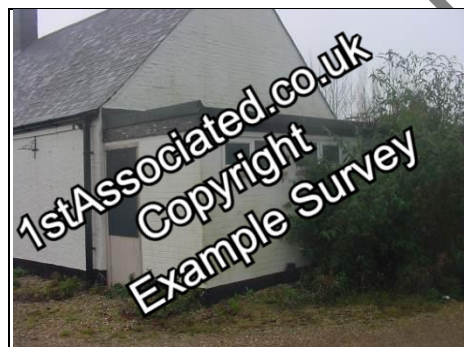
Painted Stretcher bond brickwork
