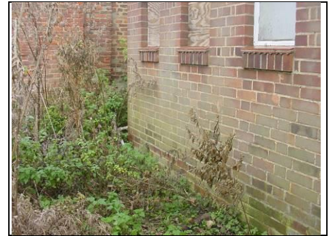
Rear of the ladies' toilets
