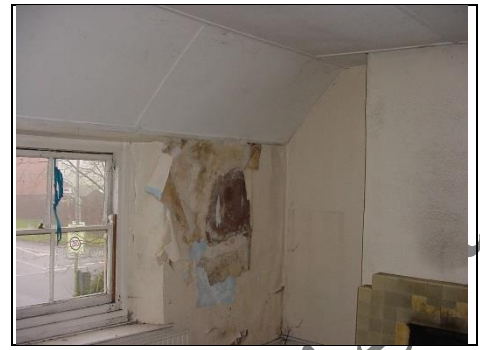
Gypsum plaster to front left ceilings
