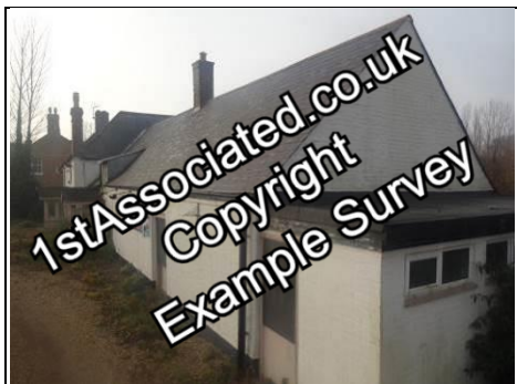
Painted Stretcher bond brickwork to the right of the property Aerial view – 360 photo
