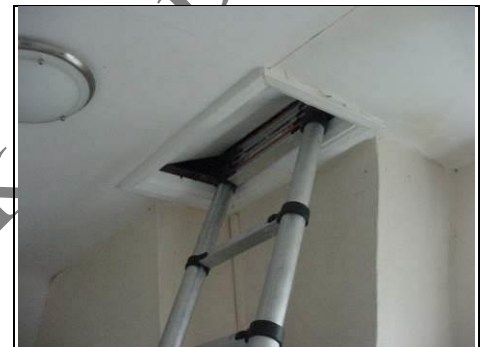
Loft hatch in the shower room
