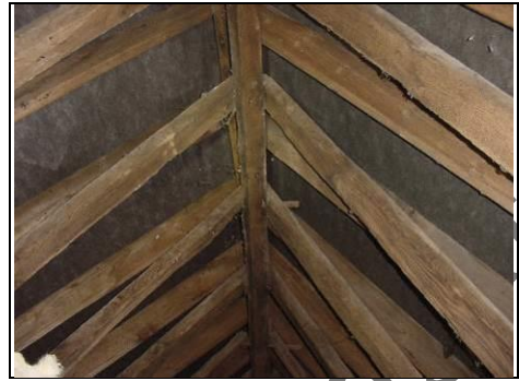
General view of inside of roof
