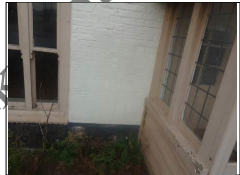
Painted brickwork Aerial view – 360 photo
