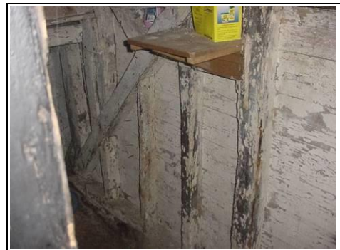
Lime washed timbers – this is how the timbers would have originally been
