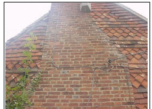
Chimney one – wrongly repointed in a cement mortar
