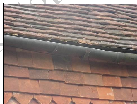
This gutter does not look to have a fascia board
