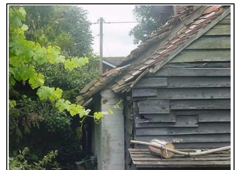
Shiplap boarding deteriorating
