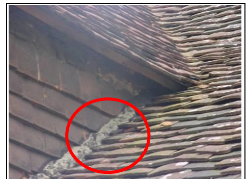
Cement flashings rather than lead flashings
