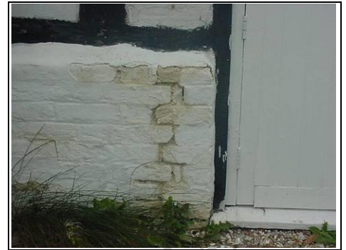
Brick plinth underneath the timber frame
