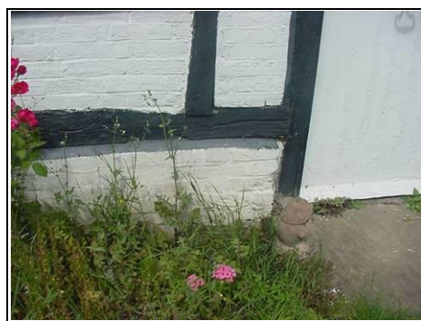
External timber frame with brick infill panel
