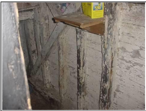
Lime washed timbers – this is how the timbers would have originally been
