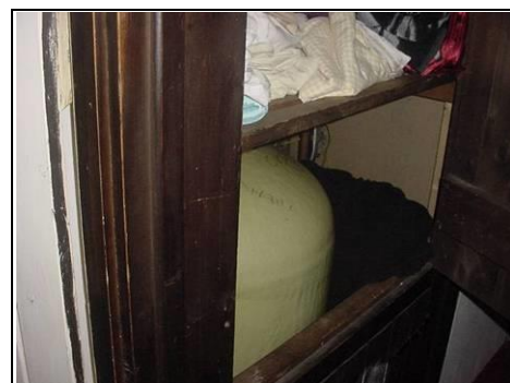
Hot water cylinder which is factory lagged
