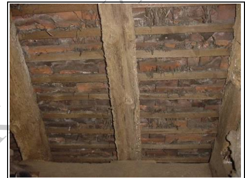
No protective underlayer (no sarking felt)
