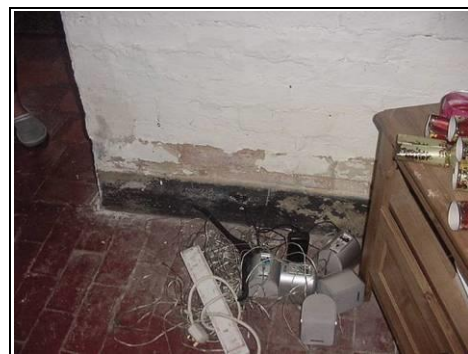
Lots of rising damp – paint coming off, we believe this to be a plastic based paint
