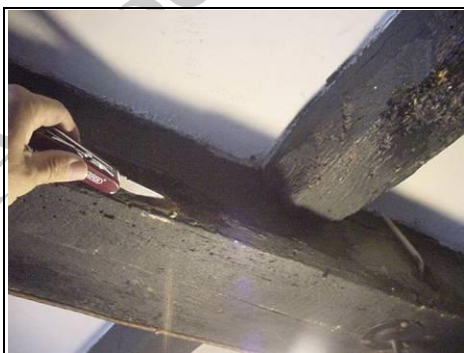
Internal spine beam with newish frass
