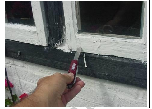
Knife testing the window
