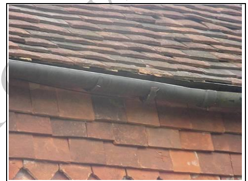
Plastic guttering
