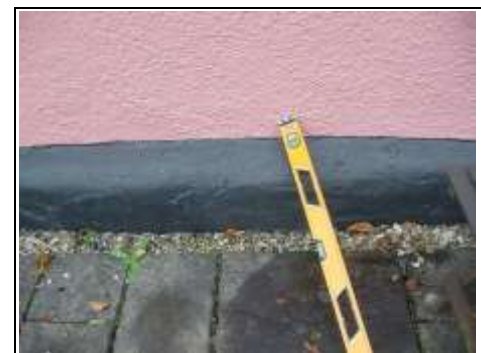
Plinth may be hiding original sole plate
