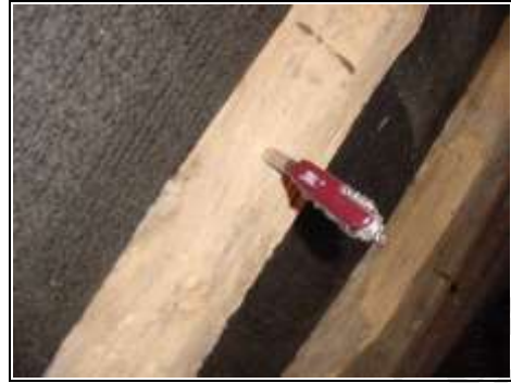
Knife could go far into roof
