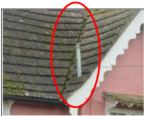
Original concrete tile valley gutter still present in some parts of the property
