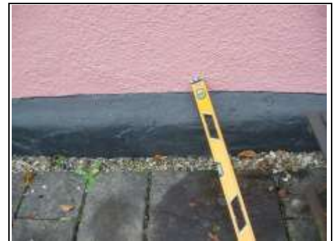
Ledge may be hiding original sole plate
