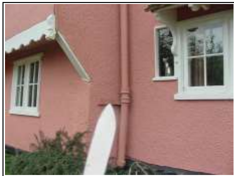
Asbestos downpipe
