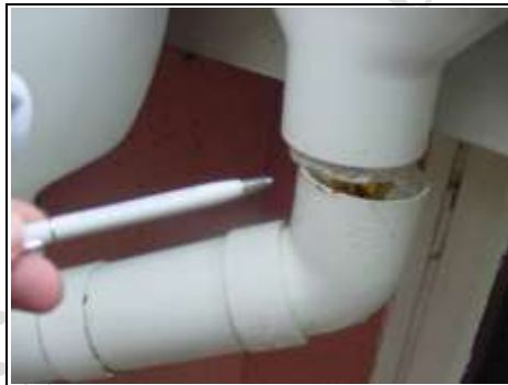
Downpipes are not fixed properly or have not been checked
