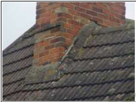
Repairs with cement and tile on edge flashing
