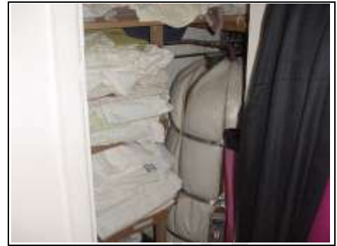
Older style hot water cylinder
