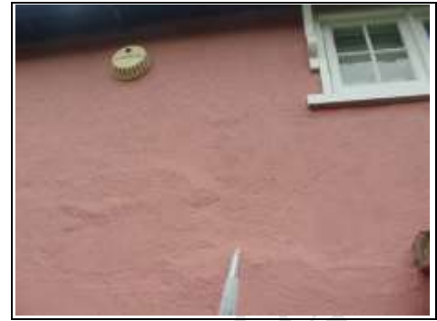
Hairline cracking
