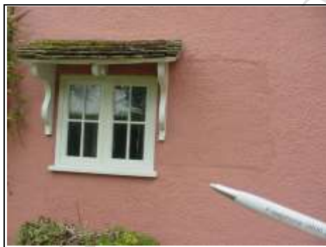
Render changes with alterations that have happened over the years
