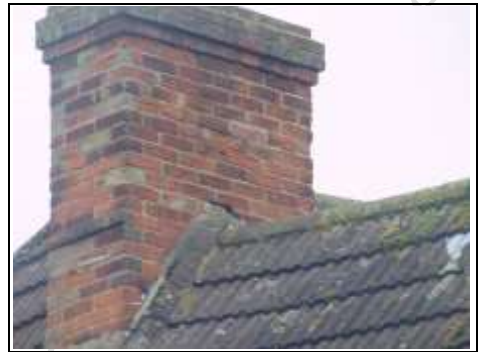
Repairs in cement and weathered
