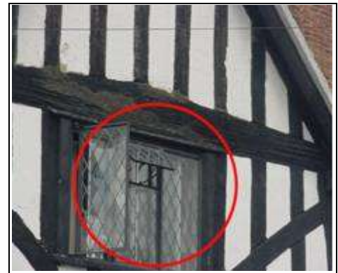
Old style diamond panel lead light in cast iron window opened to air room
