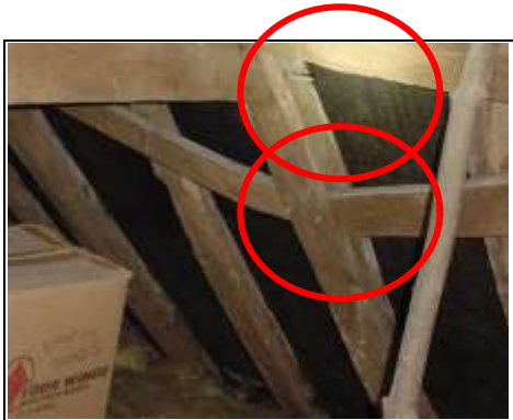
Main roof coupled with peg fixing
