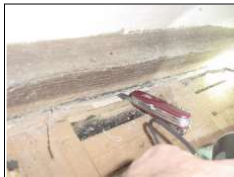
Knife going into sole plate
