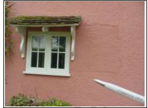
Render changes with alterations that have happened over the years
