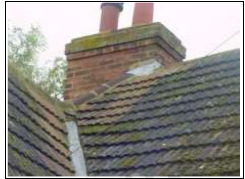
Replacement valley gutter to front left side which current owner carried out
