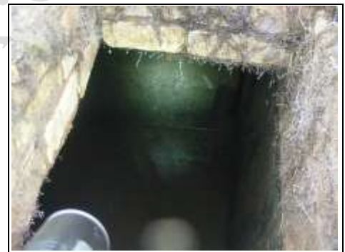
Minor roots visible in septic tank
