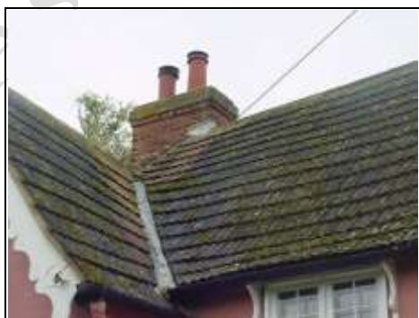
Concrete tile roof
