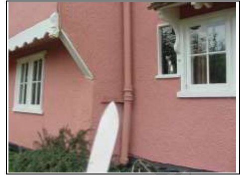
Asbestos downpipe
