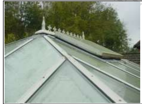
Conservatory roof starting to moss over
