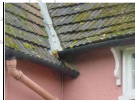
Lead valley gutter. Will it overflow the guttering?
