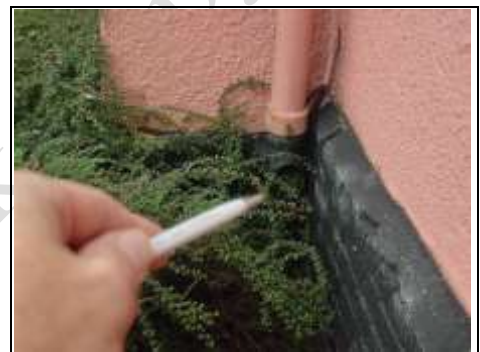
Downpipe discharging onto ground against building
