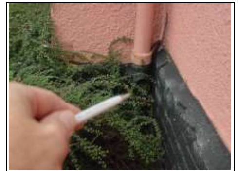
Downpipe discharging onto ground against building
