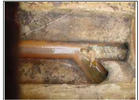
Shallow drain close to front of property
