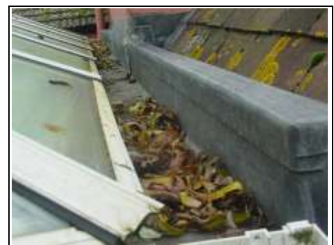
Leaves in hidden box gutter to rear
