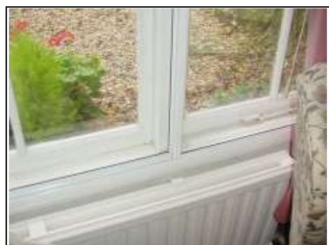
Secondary glazing to many of the windows
