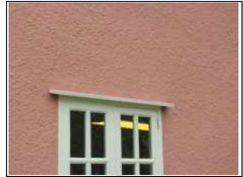
Timber drip detail
