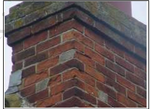
Cement repairs
