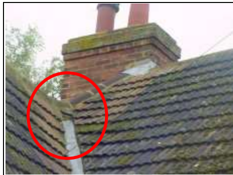
Lead valley gutter added. Note: Tiles have been repaired
