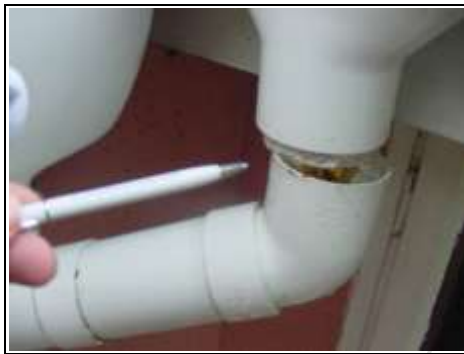
Downpipes are not fixed properly or have not been checked
