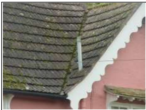
Soil and vent pipe
