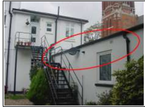
Converted Georgian flats extended to the rear
