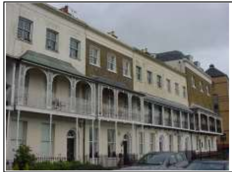
Regency properties with iron work detail
