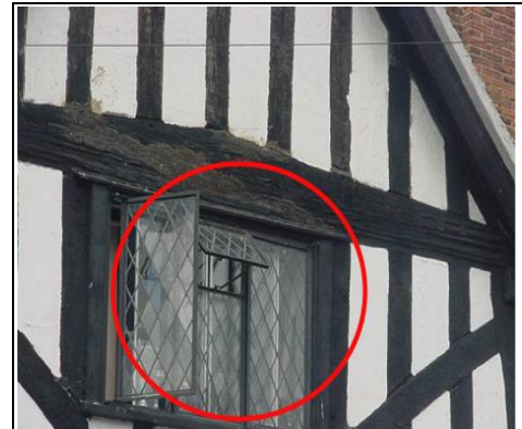
Tudor property with old style diamond panel lead light in a cast iron window. This is one of the earliest windows outside of the church, royalty and other wealthy establishments
