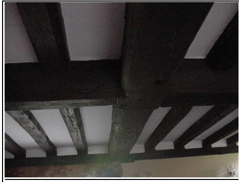
Timber frame ceiling
