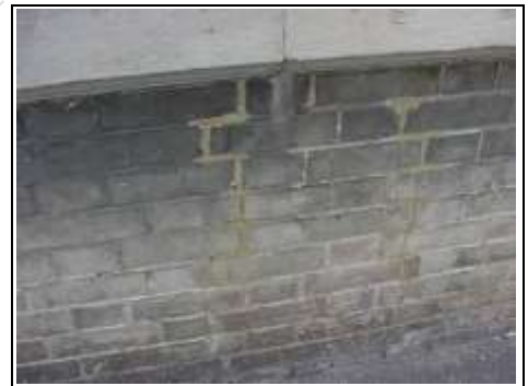
Repairs to cracking
