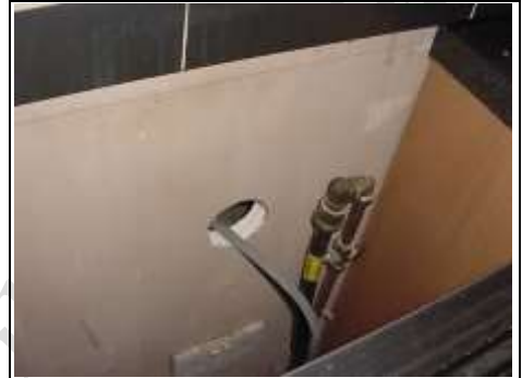
False wall / dry lining in the kitchen
