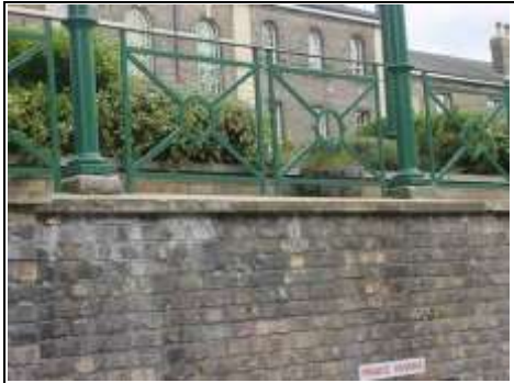
Retaining wall without weep holes
