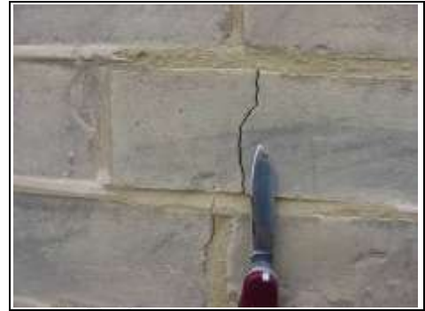
Vertical crack in the brickwork
