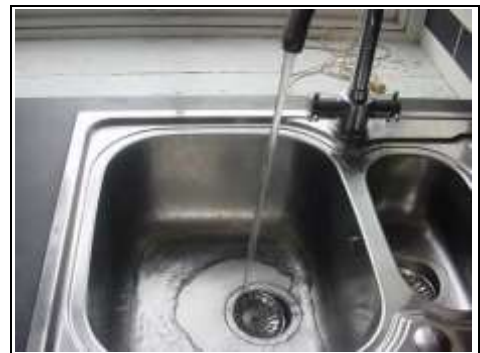
Taps run for 15 minutes to check for blockages
