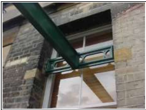
Unusual window with cast iron beam
