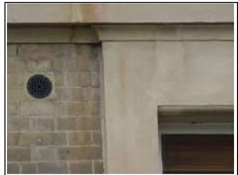
Vent for the gas boiler
