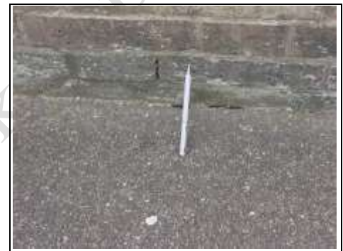
Damp proof course is too low for the ground level
