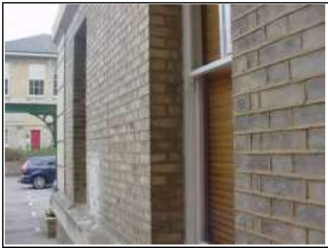
Re-pointing carried out in cement and not lime
