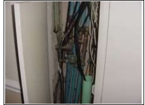
Plastic and copper pipe in communal area
