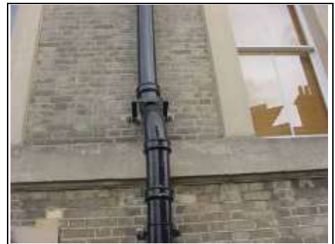
Possible asbestos downpipes
