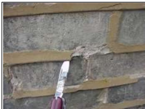
Poor re-pointing. Just a skim coat we are amazed it has stayed on.
