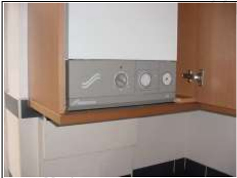
Wall mounted Worcester Boiler
