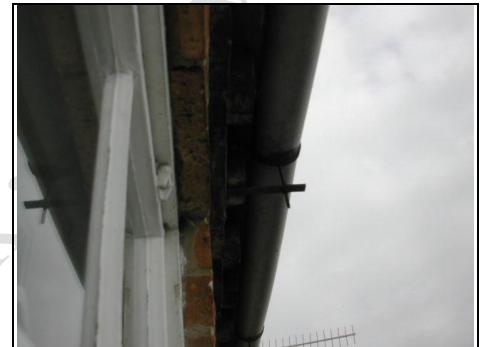
Plastic gutter to rear elevation
