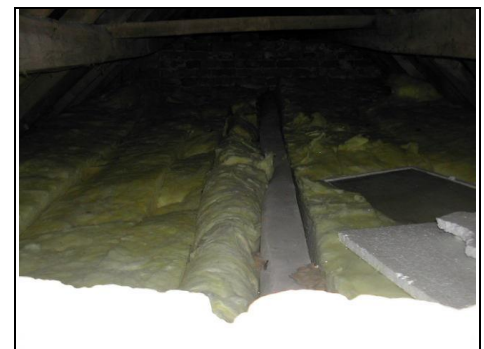
Rear roof pitched area
