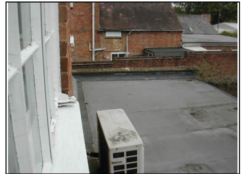
Parapet to flat roof
