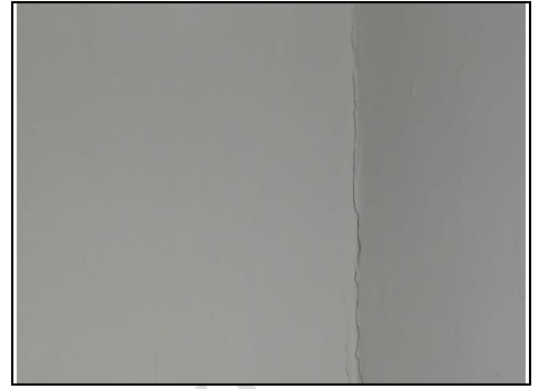
Wall cracks
