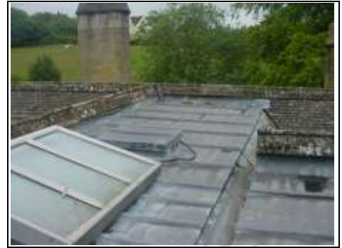
Rolled lead flat roof
