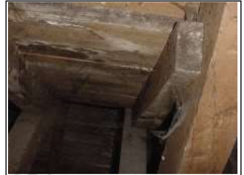
Dampness in timbers to valley gutters
