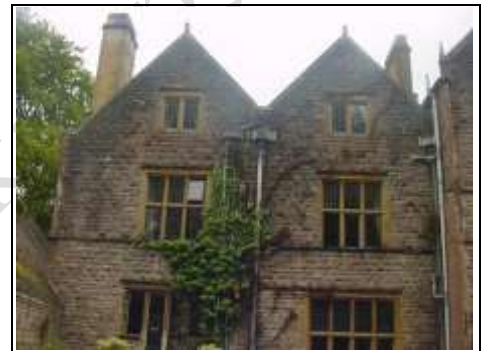
Plants growing over soil and vent pipes and also the downpipes
