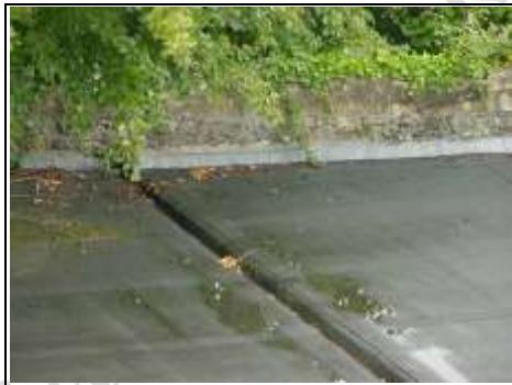
Central drain to flat roof
