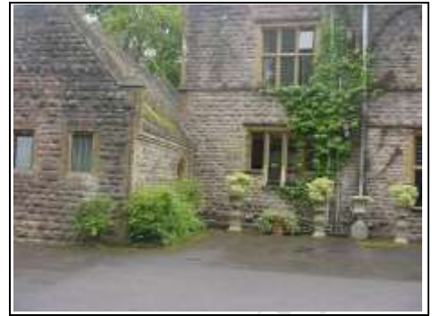
Tarmac passing surface water towards the property
