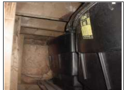
Dampness directly above the water tank
