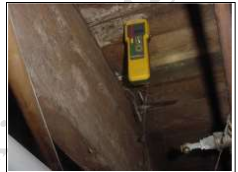
Dampness coming through the flat roof below the lead work
