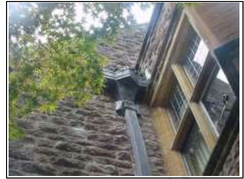
Looking up at a lead hopper head and downpipe and surrounding trees
