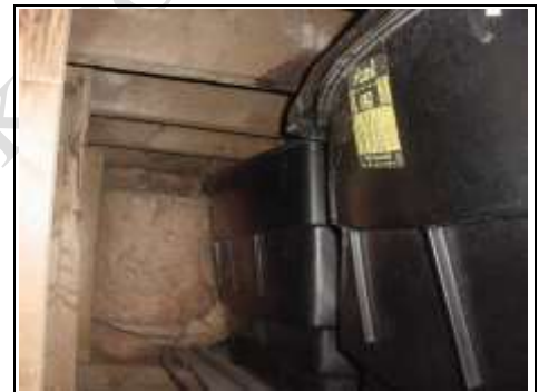
Looking at dampness beneath flat roof that has condensation from the water tanks
