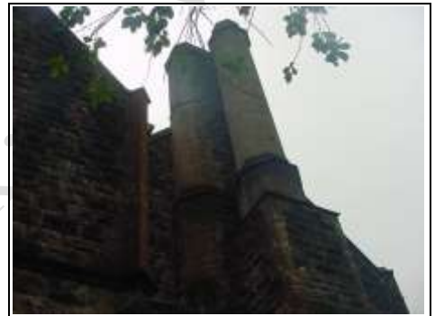
Rear right hand chimney which is starting to deteriorate
