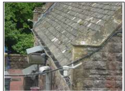
Lead gutter on left hand side of building
