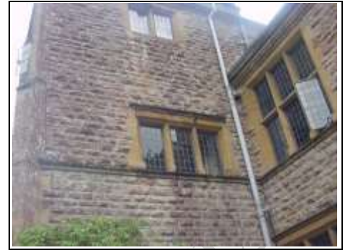
Plastic soil and vent pipe
