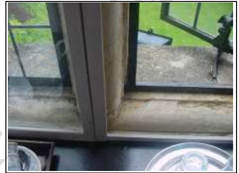
Windows deteriorating
