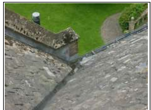
Valley gutter that is becoming blocked next to a lead guttering
