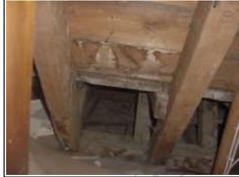
Far right hand side – we could see some water staining indicating that dampness was getting through
