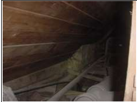
Far left hand side – here you can see a timber decking has been used to support the valley gutter which looks in reasonable condition
