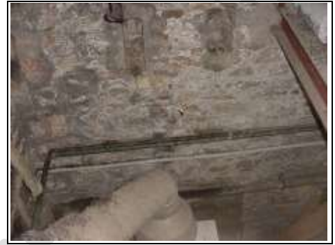
Asbestos going down to boiler in handyman's room and boiler room
