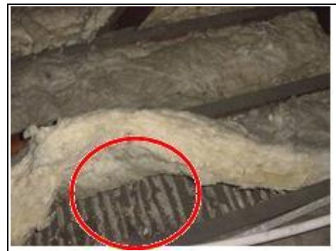
Lath and plaster
