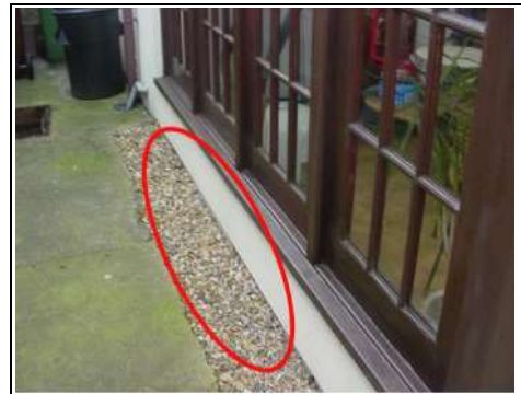
French drain under shingle
