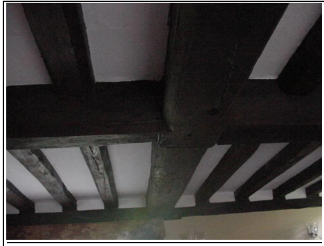
Timber frame ceiling
